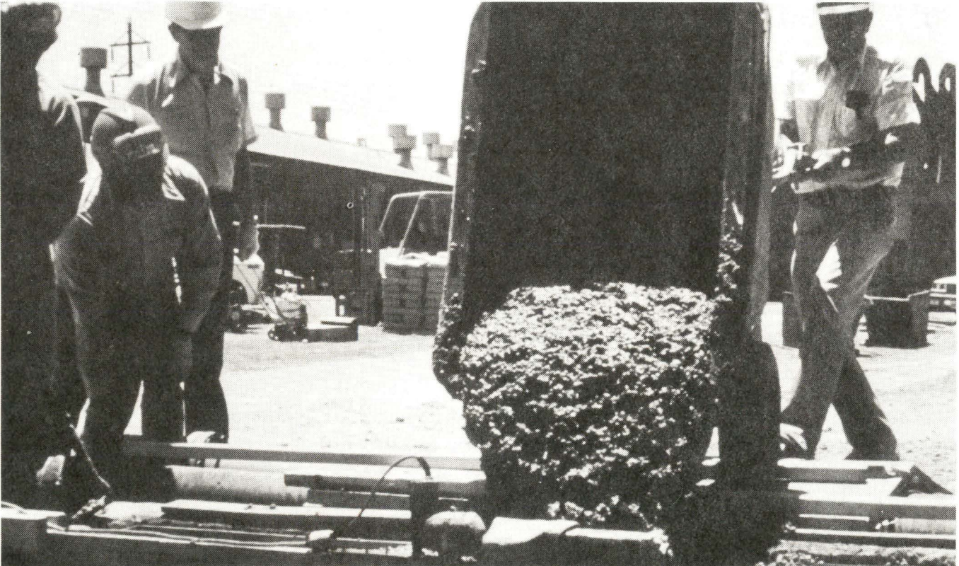
FIGURE 21. - Pouring a sulfur concrete floor.
