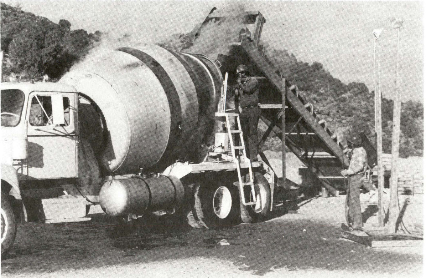
FIGURE 22. - Sulfur concrete preparation in a heated concrete mixer.
