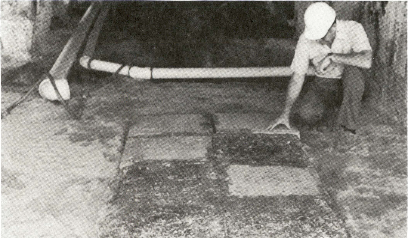
FIGURE 20. - Sulfur concrete test slabs in electrolytic zinc plant.
