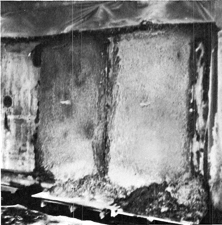
FIGURE 3. - Completed shotcrete panels.
