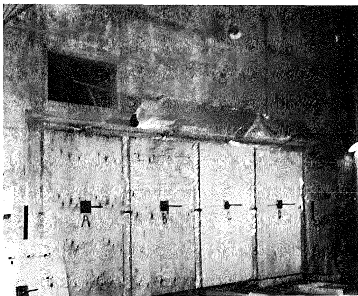
FIGURE 2. - Mounted plywood panels.
