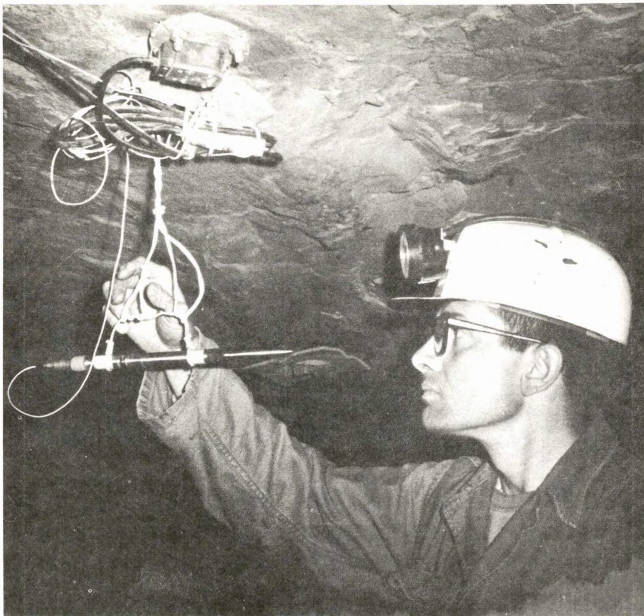
FIGURE 3. - Alinement of Blast Pressure Gage in Haulageway.
