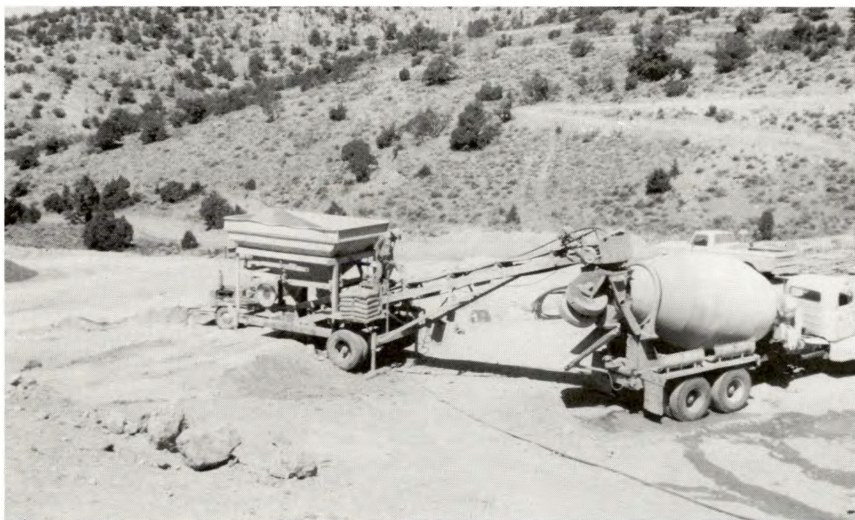
FIGURE 10. - Batch agglomeration equipment from pilot-scale experiment conducted near Ely, Nev.
