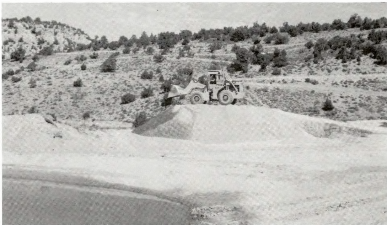
FIGURE 11. - Heap (2,500 tons) agglomerated with cement and cyanide solution under construction near Ely, Nev.
