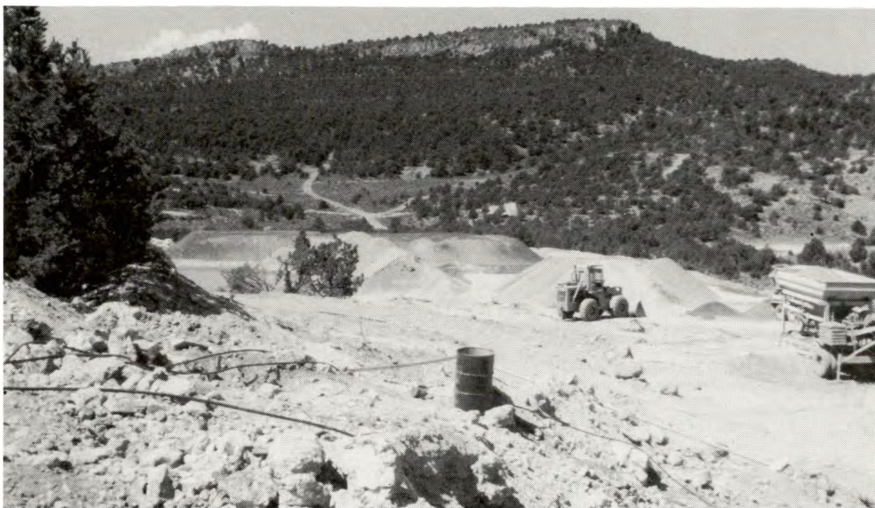
FIGURE 9. - Overall view of pilot-scale agglomeration experiment conducted on gold ore from near Ely, Nev.
