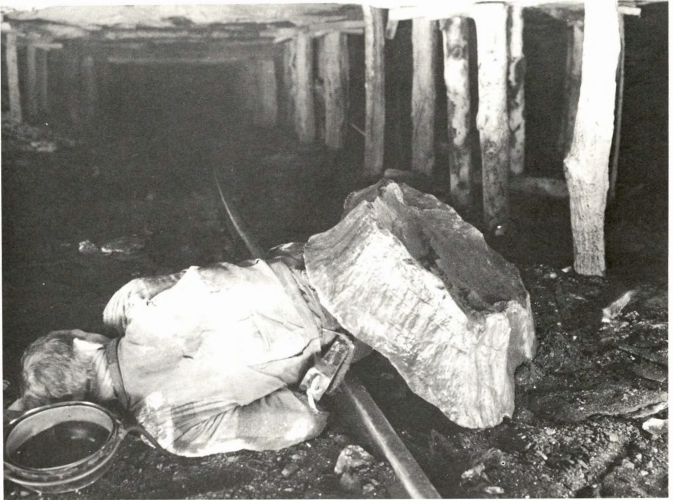
FIGURE 1. - Illustration of the hazards posed by fall of a kettle bottom.
