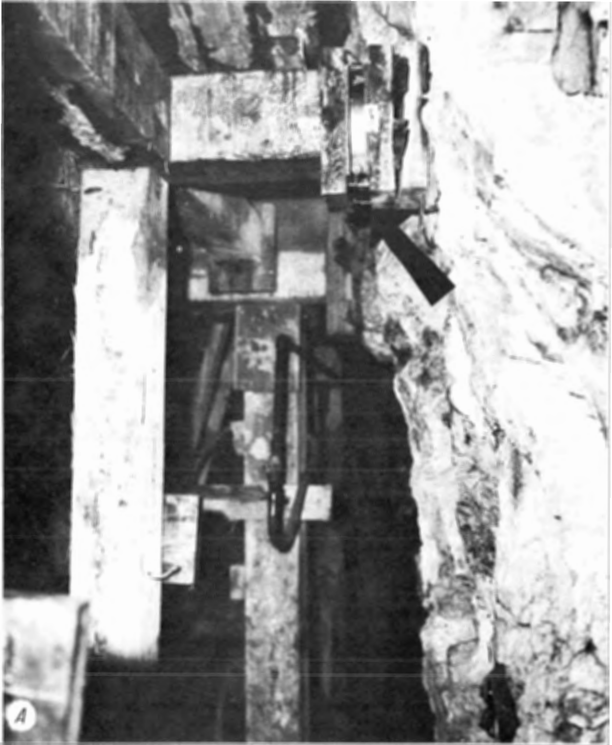
FIGURE 22. - Field test of load cells in a "hardrock" mine. A , Flat-compression load cell installed in a cap set; B , rock-bolt load cell installed on 6-foot, 3/4-inch rock bolt.
