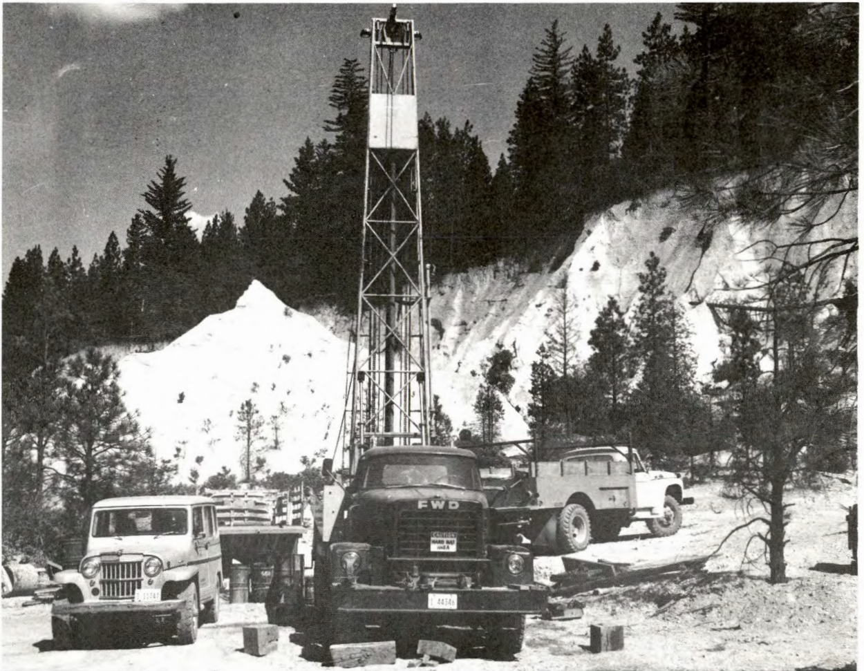
FIGURE 19. - Rotary drilling in cemented gravel.
