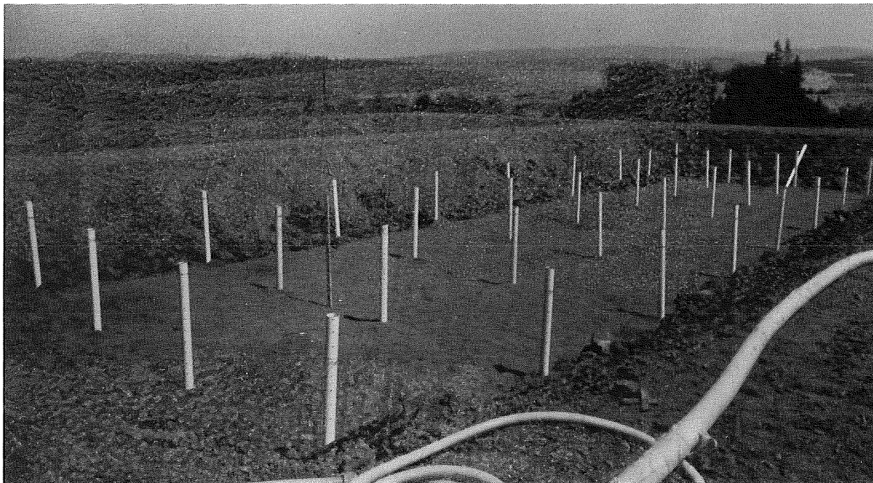
FIGURE 6. - Vertical sand drains.
