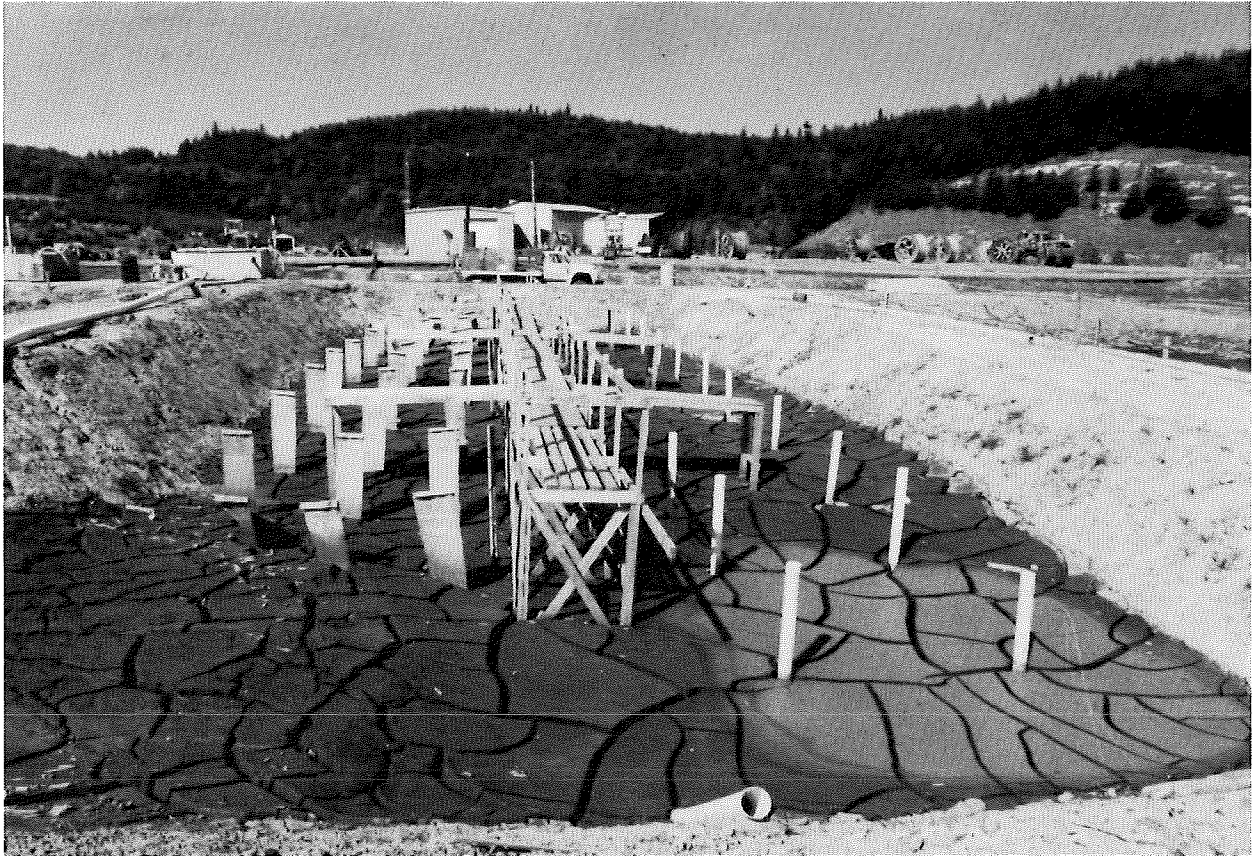
FIGURE 10. - Test cell with vertical sand and fabric drains.
