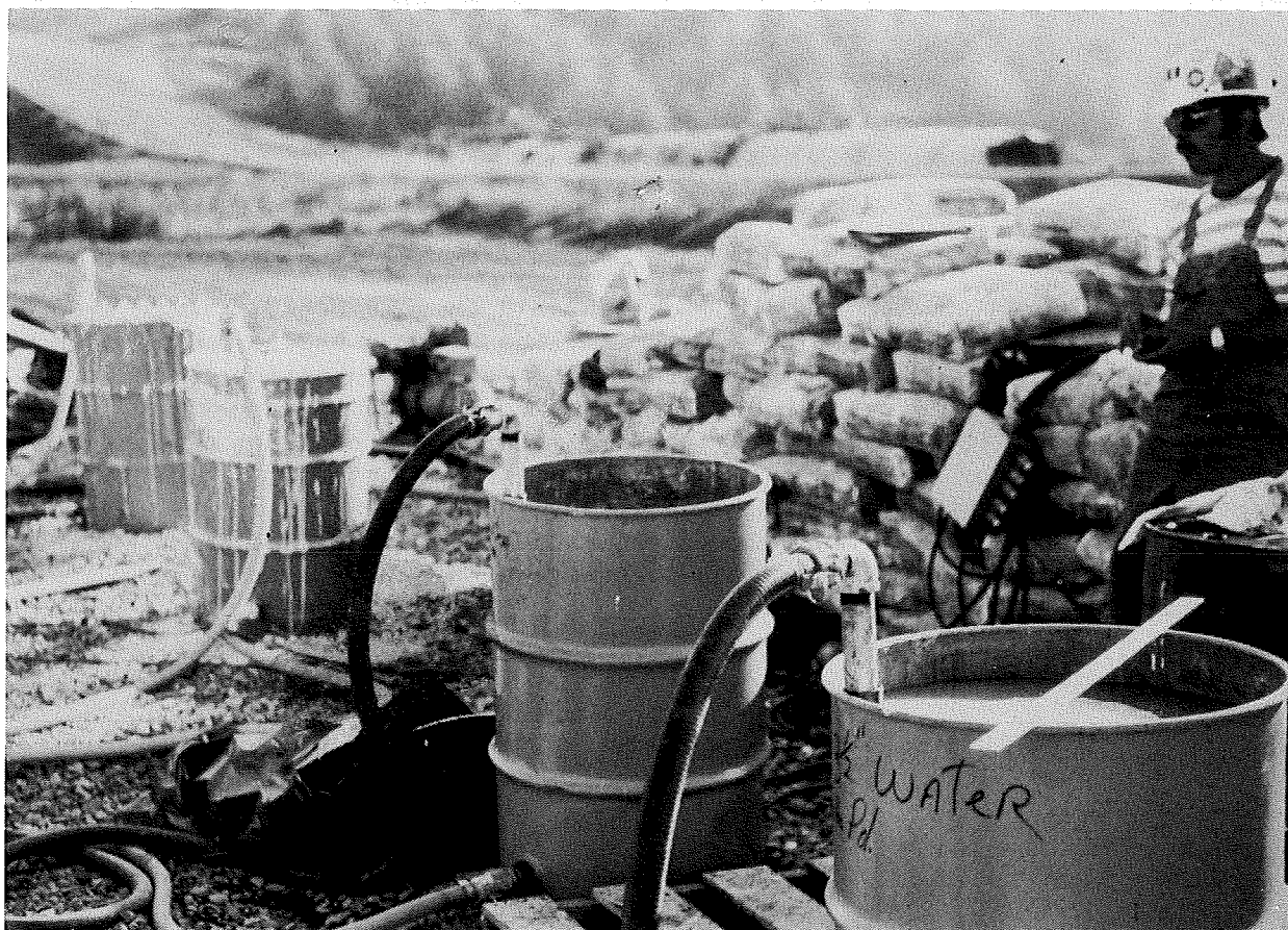
FIGURE 2. - Chemical treatment mixing drums.
