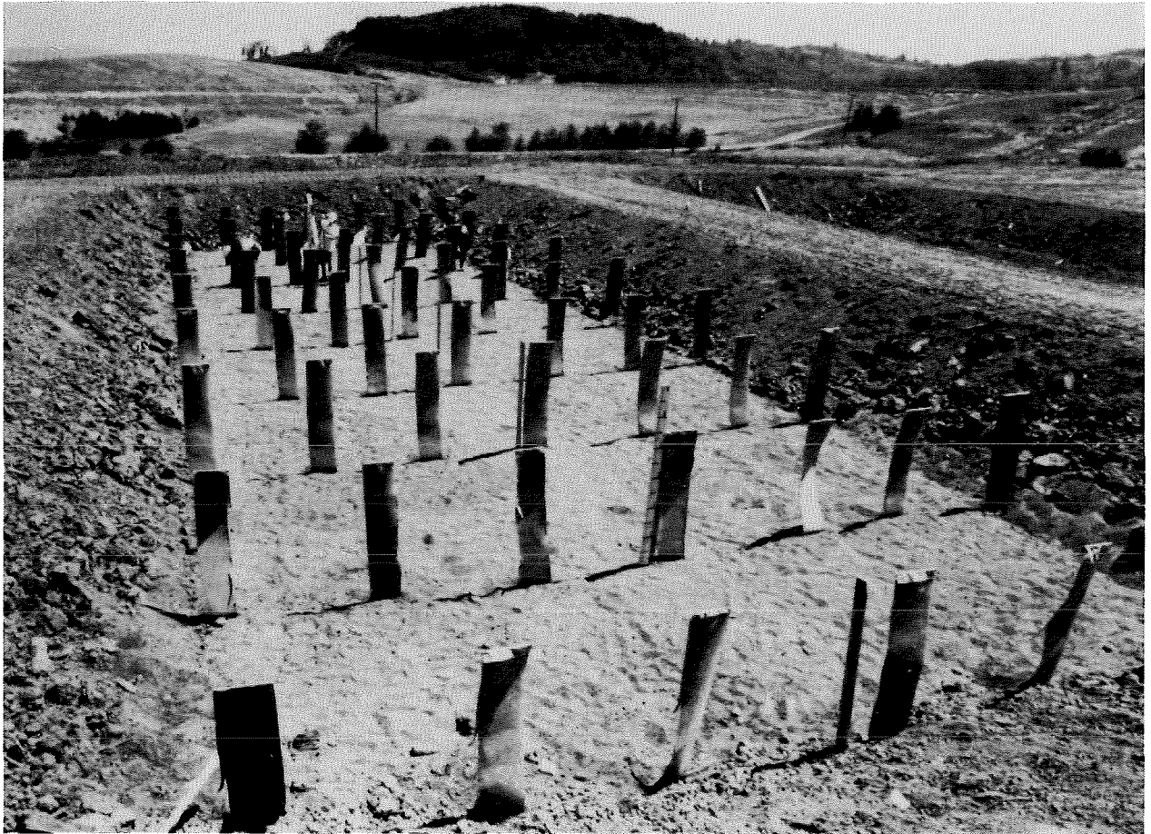
FIGURE 7. - Vertical fabric drains.
