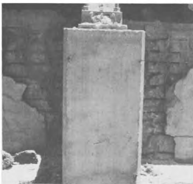
Figure 15.—Corrosion of PCC by acid electrolytes in electrolytic zinc plant.
