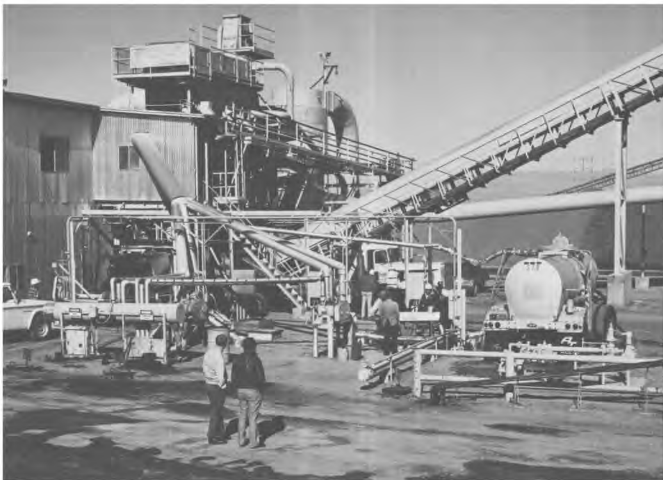
Figure 44.—Modified asphalt mix plant for preparing SEA pavement using direct-mix method.
