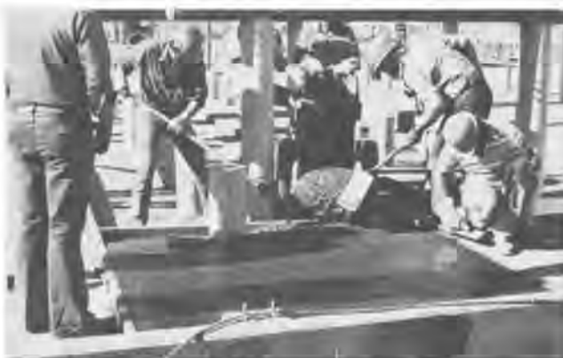
Figure 20.—Installing SC floor in electrolytic copper plant.
