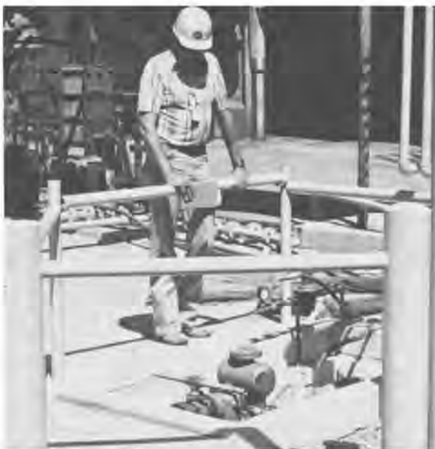
Figure 18.—SC pump support unit installed with a chlorine gas pump.
