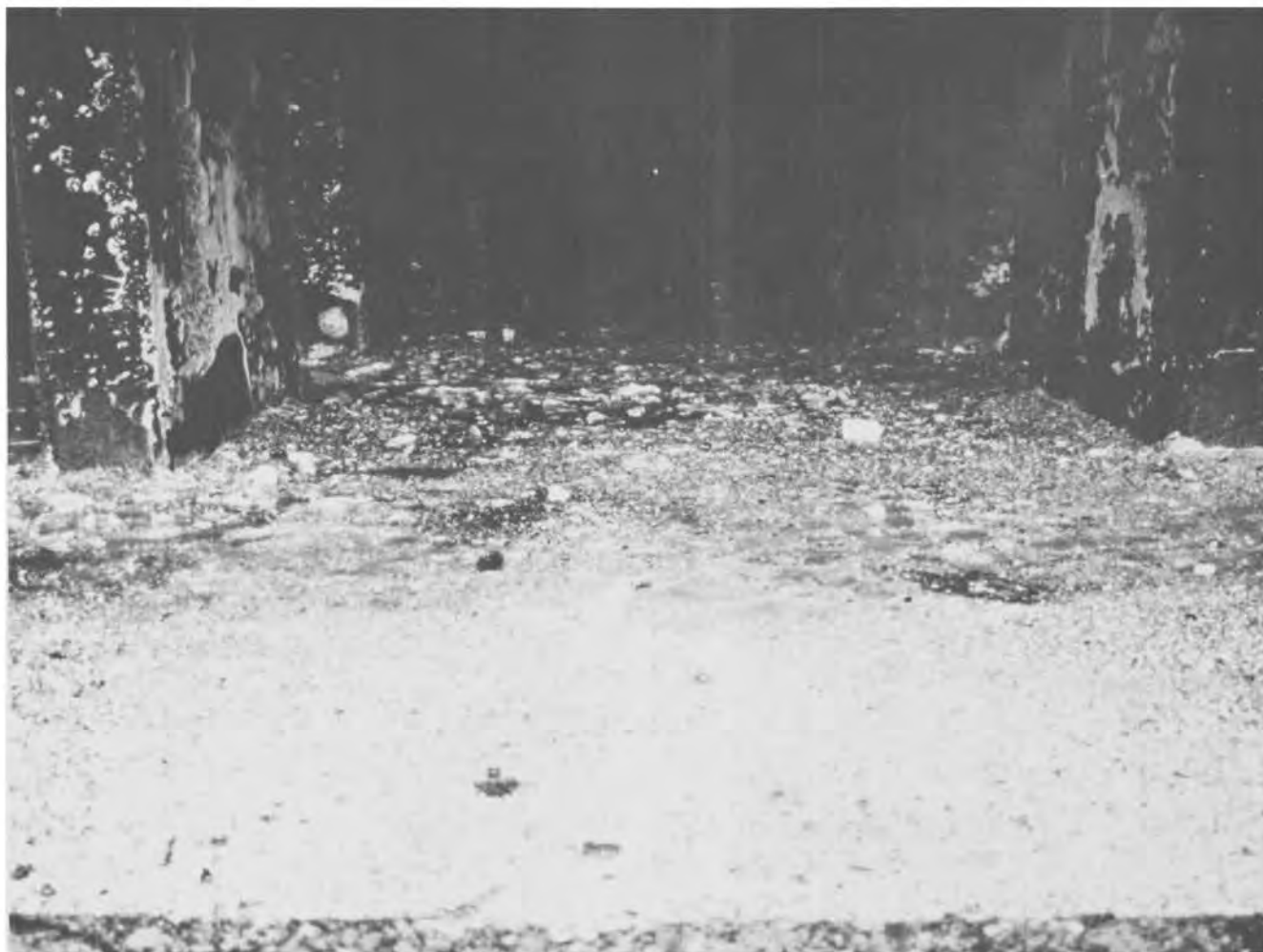
Figure 15.—Corrosion of PCC by acid electrolytes in electrolytic zinc plant.
