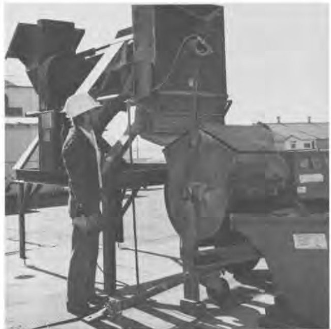
Figure 21.—Small-scale (500-lb) batch plant for SC.
