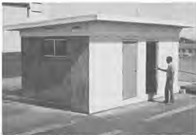
Figure 26.—Surface-bonded block building.
