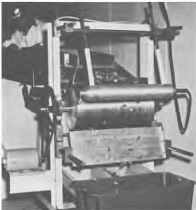
Figure 32.—High-tension (electrodynamic) separator used to separate paper from plastic.
