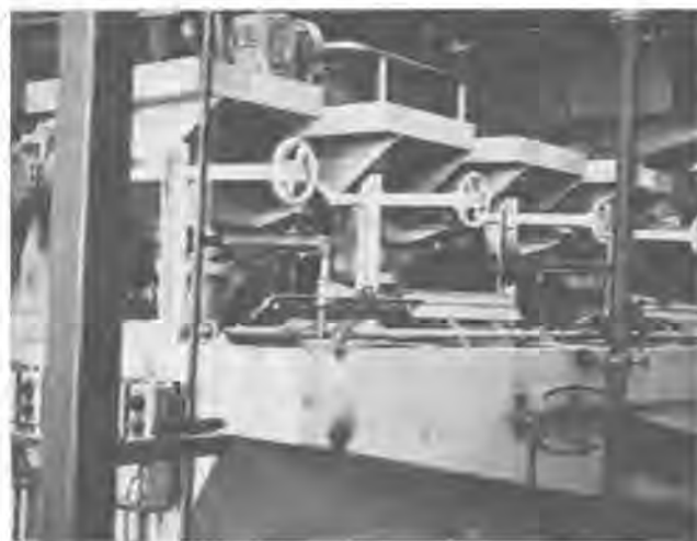
Figure 34.—Froth flotation cells for recovering glass at the Delaware Solid Waste Authority Reclamation Plant.
