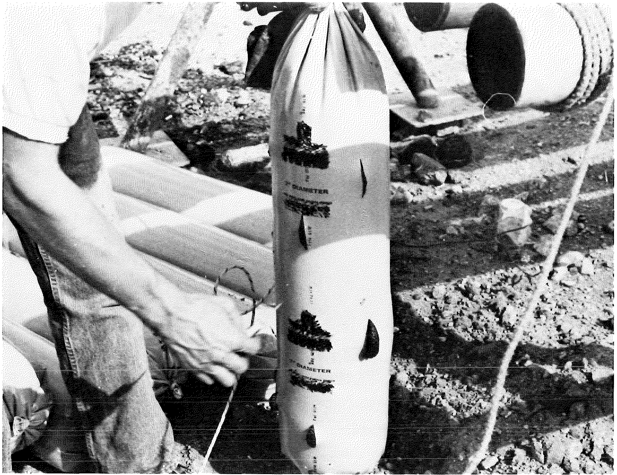
FIGURE 11. - Cutting 50-pound bags of slurry before lowering into blastholes.
