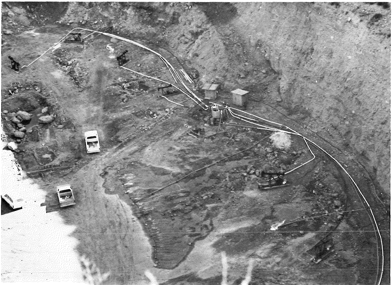
FIGURE 32. - Pit area during pit bottom leaching.
