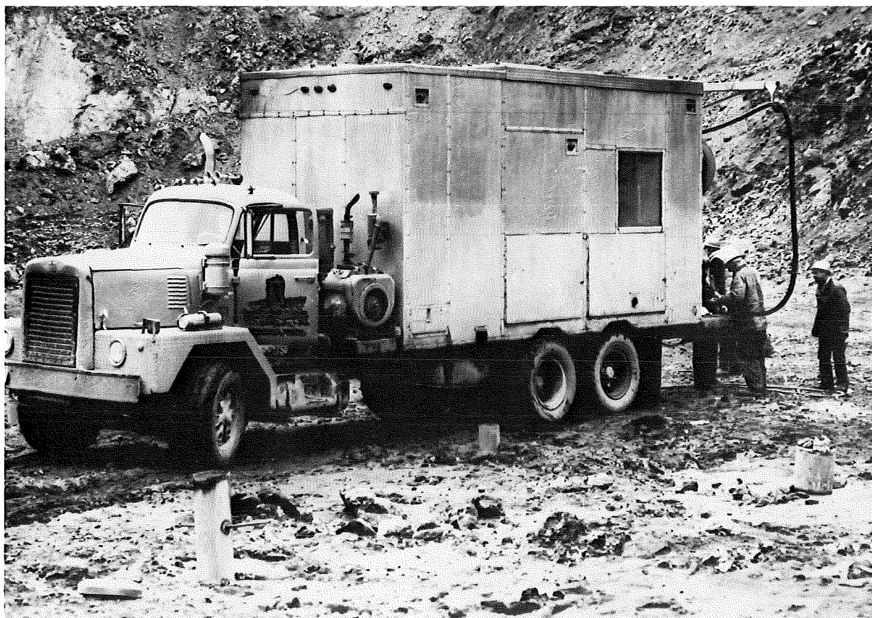
FIGURE 10: - Phase I blasthole loading.
