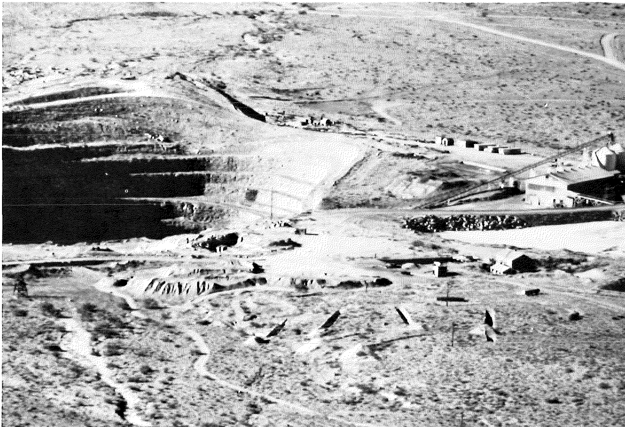
FIGURE 3. - A view of the Emerald Isle mine looking west.
