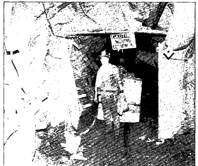
Figure 31.—Hanging wall drift on 3650 level showing buckling of old air door frame.
