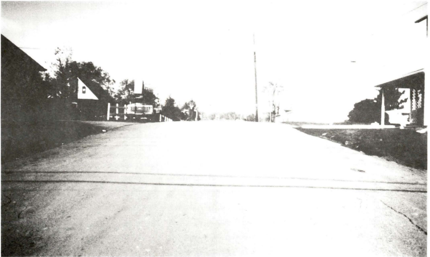
View of ground surface above tunnel, looking toward upper tunnel end. Upper tunnel end is at end of street near utility pole.
