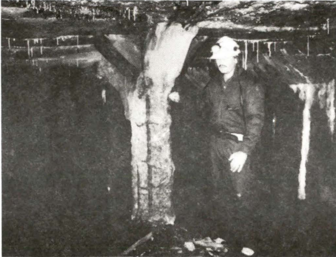
One of three concrete columns in tunnel.
