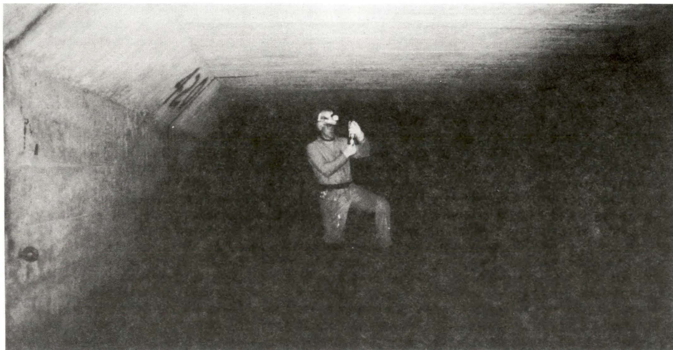
Air-quality testing in tunnel interior.
