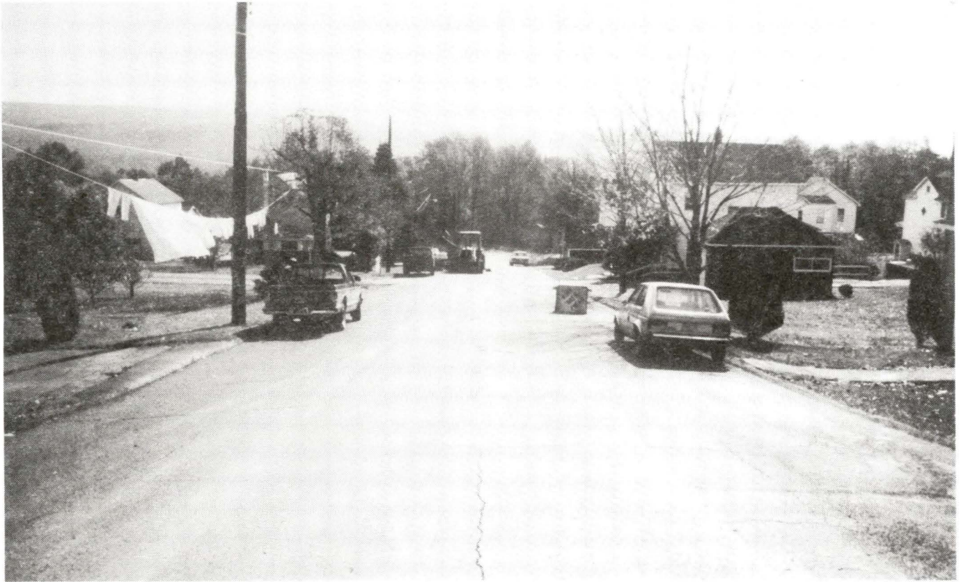
View of ground surface above tunnel, looking toward lower tunnel end. Lower tunnel end is at end of street near tree line.
