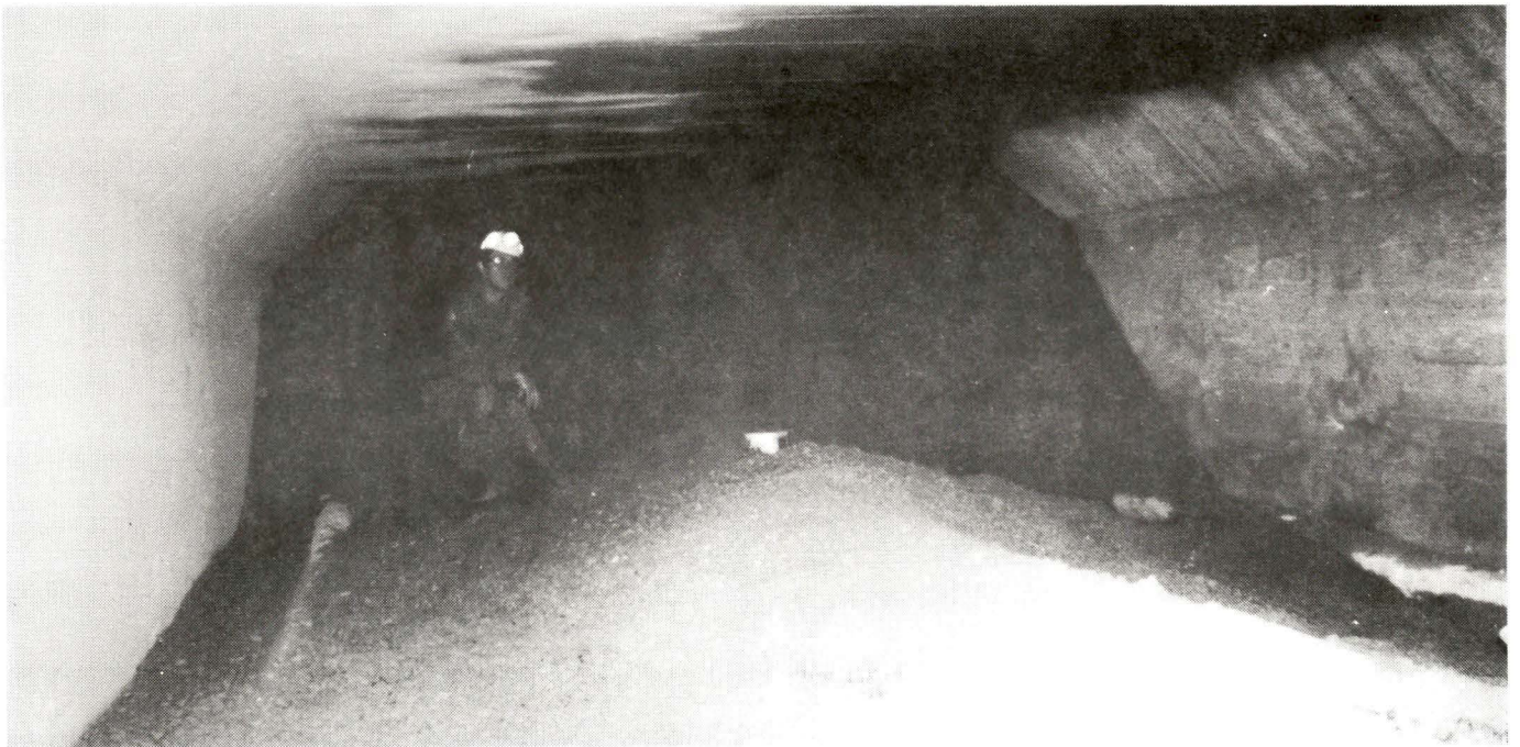
Deposition of backfill in tunnel interior.
