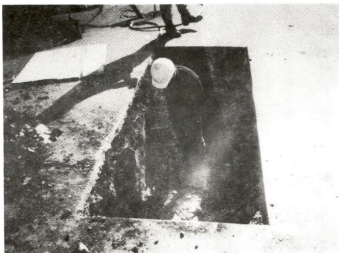
Preparation of hole 1.
