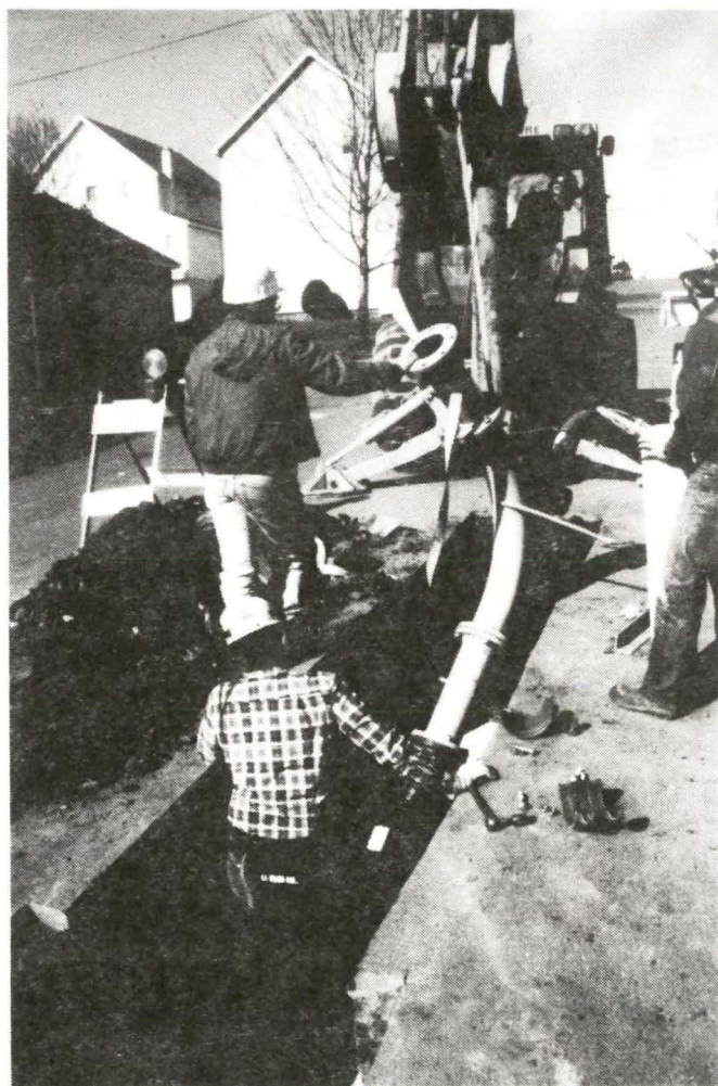
Installation of Pneumatic Pipefeeder in hole 1.
