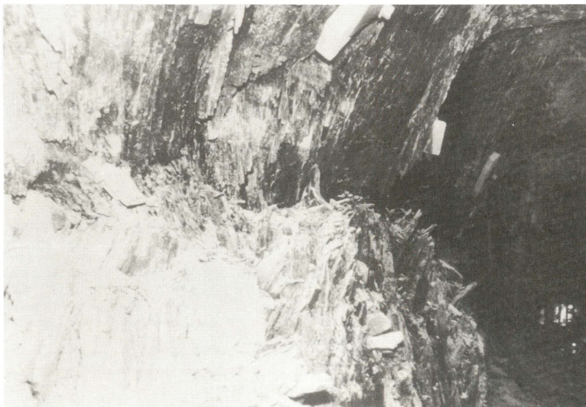
Figure 8.—Rib spalling and bolting along zone C of pillar.
