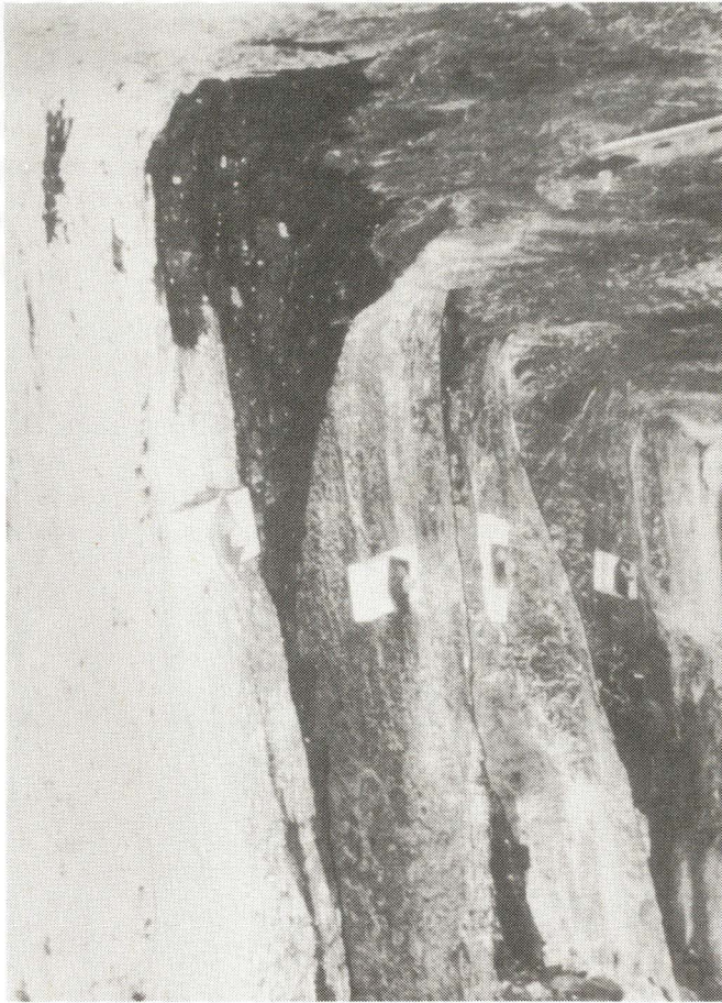
Figure 6.—Slab formation and rib bolting along zone A of pillar.
