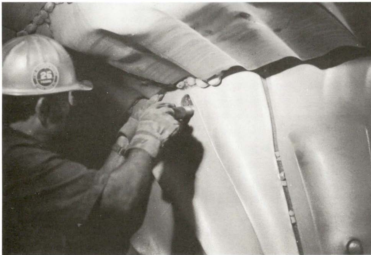
FIGURE 10.—Installation of electrode assembly in ball mill.
