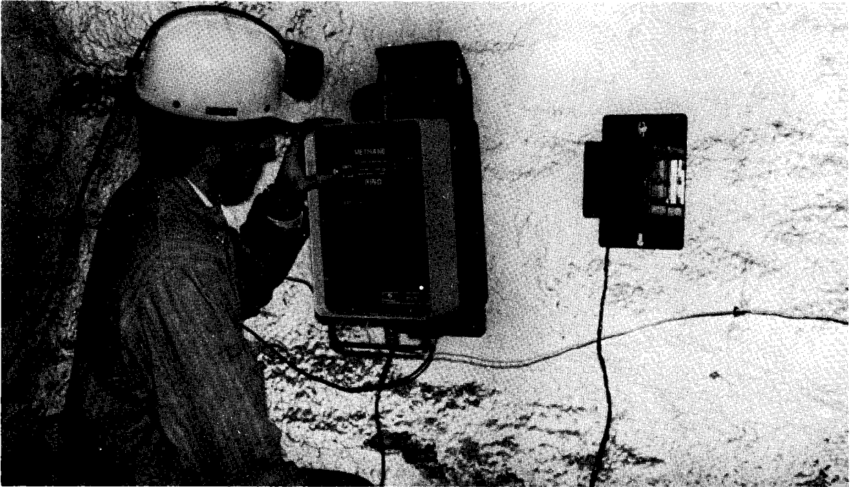
FIGURE 12. - Emergency voice receiver installed to right of escapeway phone. Miner shown activating ULF radio transmitter in phone.
