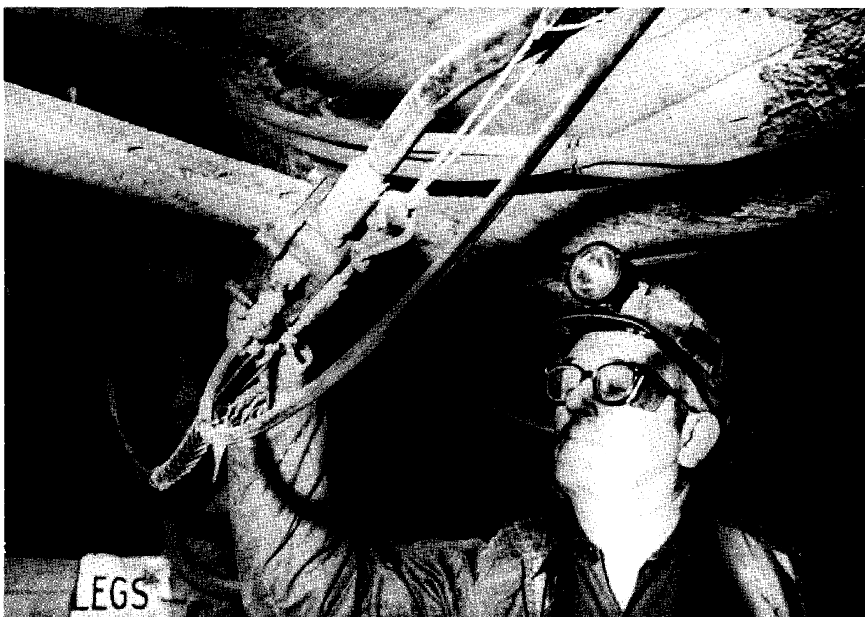
FIGURE 3. - Workman making underground phone taps.
