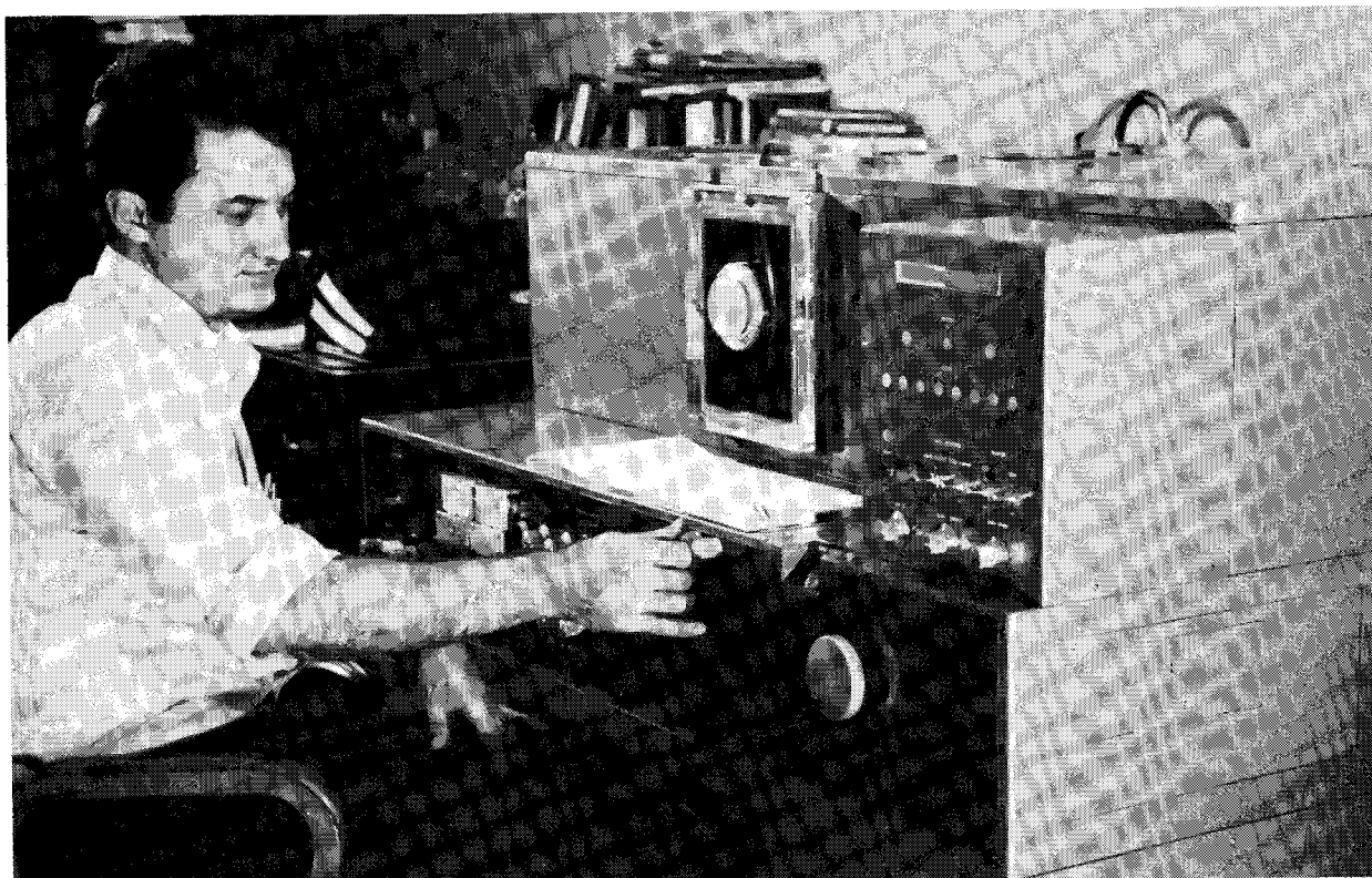
FIGURE 5. - Identifying Minerals in Coal Refuse by Far-Infrared Spectroscopy.
