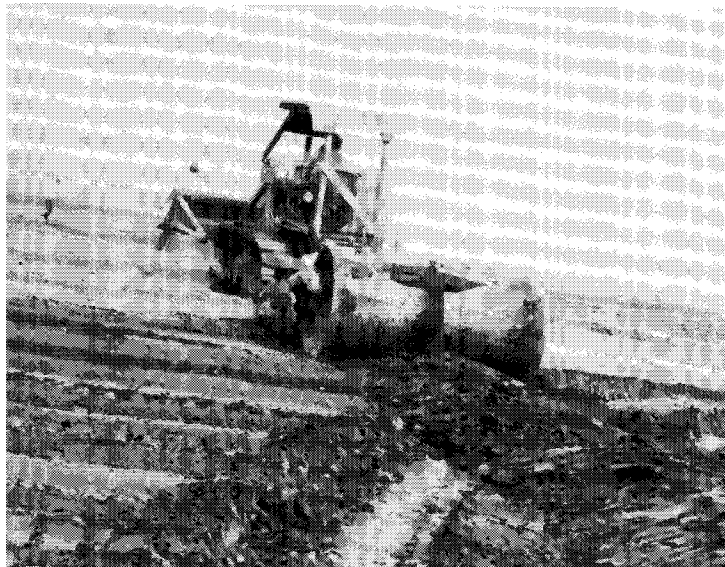
FIGURE 7. - Stabilizing Surface-Mine Spoil To Reduce Erosion and Stream Siltation.
