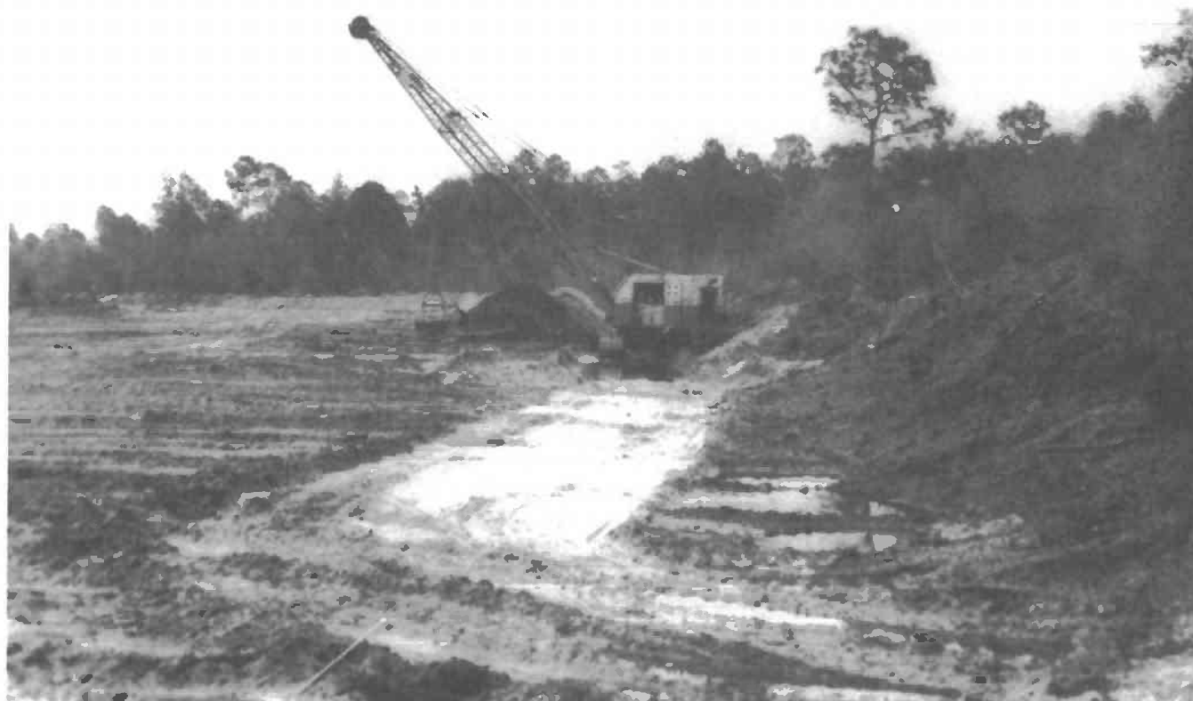
FIGURE 12.—Dike construction during test site preparation.
