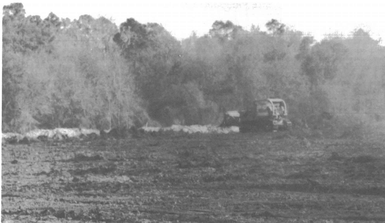
FIGURE 13.—Bulldozers clearing overstory before mining.
