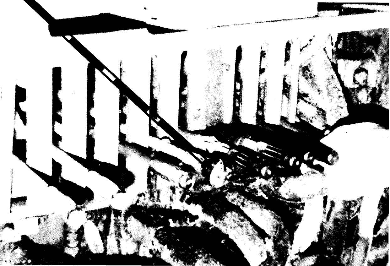
FIGURE 3. - Roof bolter controls with electrical tape to help distinguish one handle from another.
