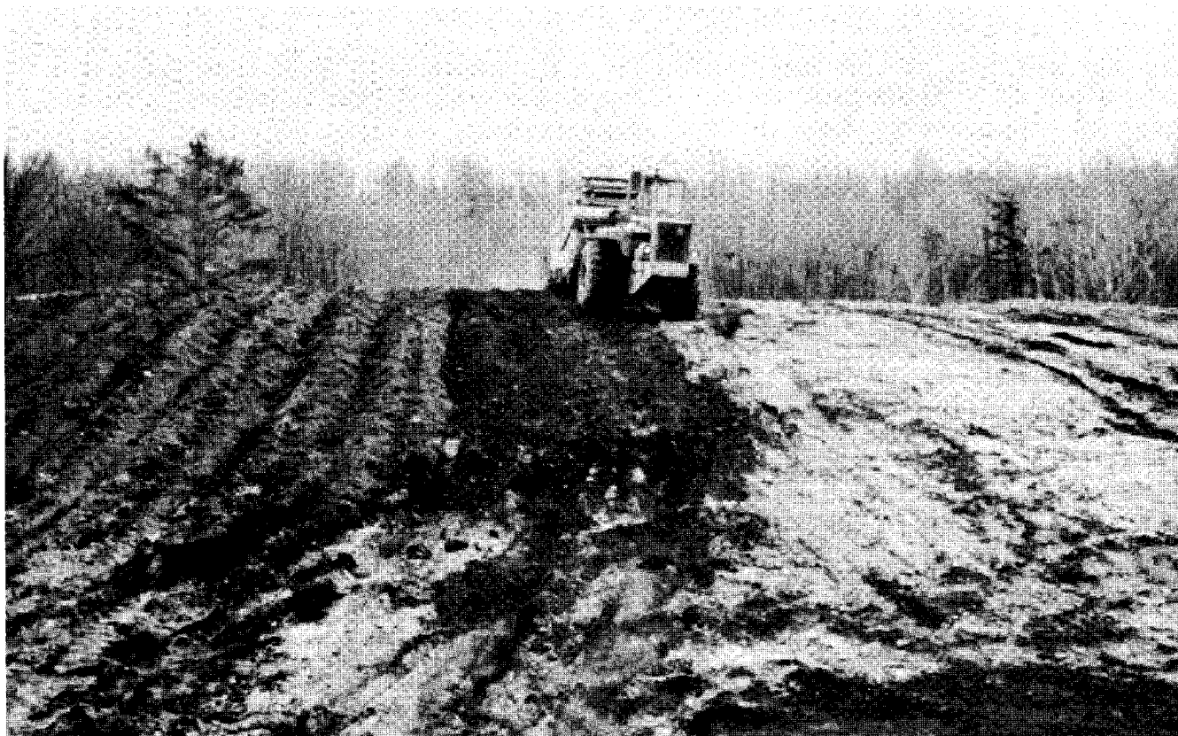
FIGURE 21. - Panther Tipple Reclamation Site. Soil preparation prior to seeding (white surface is pulverized limestone).
