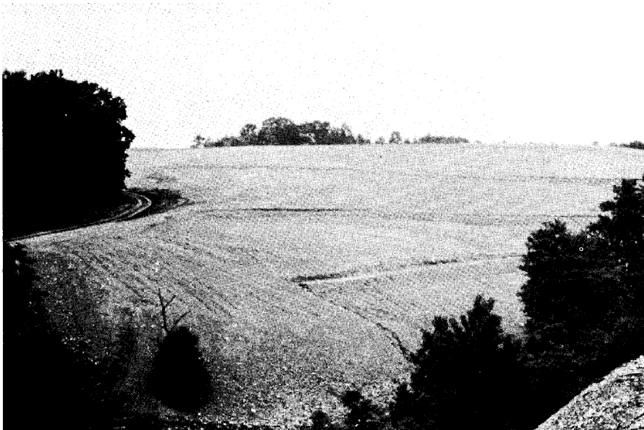
FIGURE 17. - Coal Tipple Reclamation Site. Completed reclamation showing drainage system.
