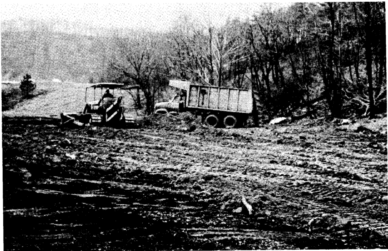
FIGURE 18. - Clymer Borough Reclamation Site. Transporting, spreading, and compacting of soil cover.
