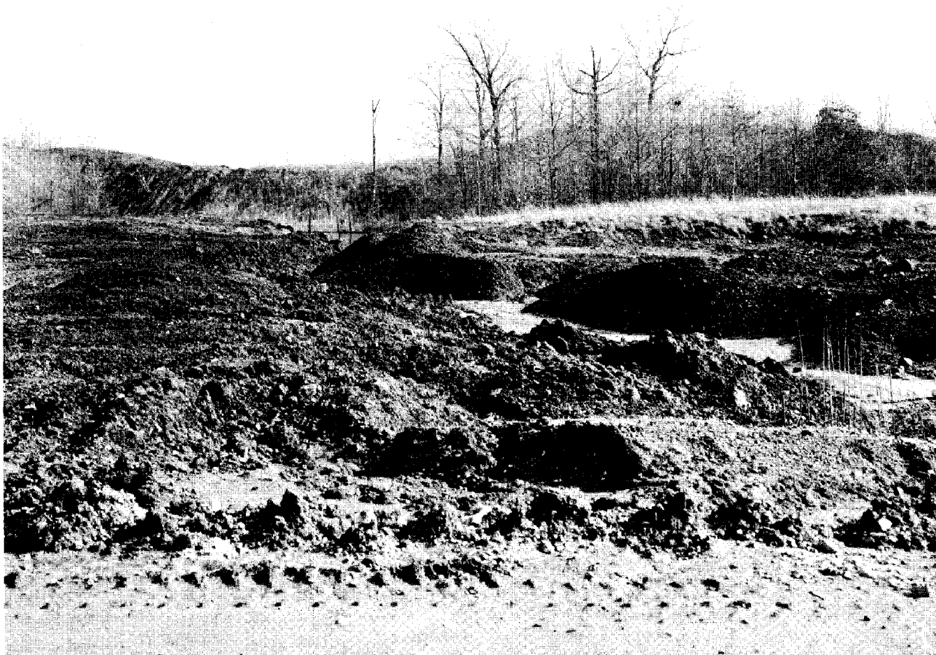
FIGURE 11. - Colonial Mine Reclamation Site. Strip mine filled with coal refuse ready for grading, covering, and planting.
