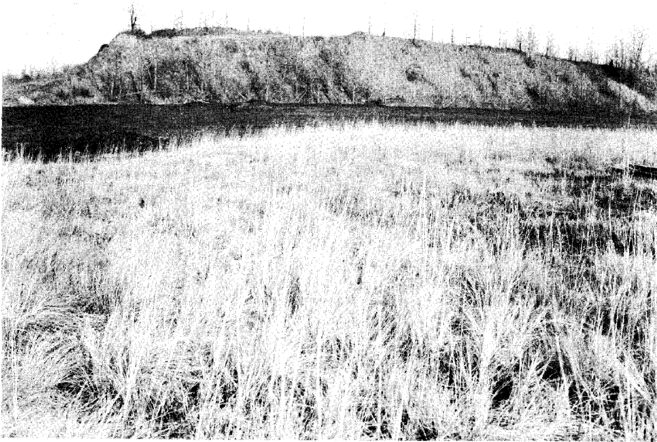
FIGURE 12. - Colonial Mine Reclamation Site. Reclaimed area in foreground. New refuse fill and soil covered bank in the background.
