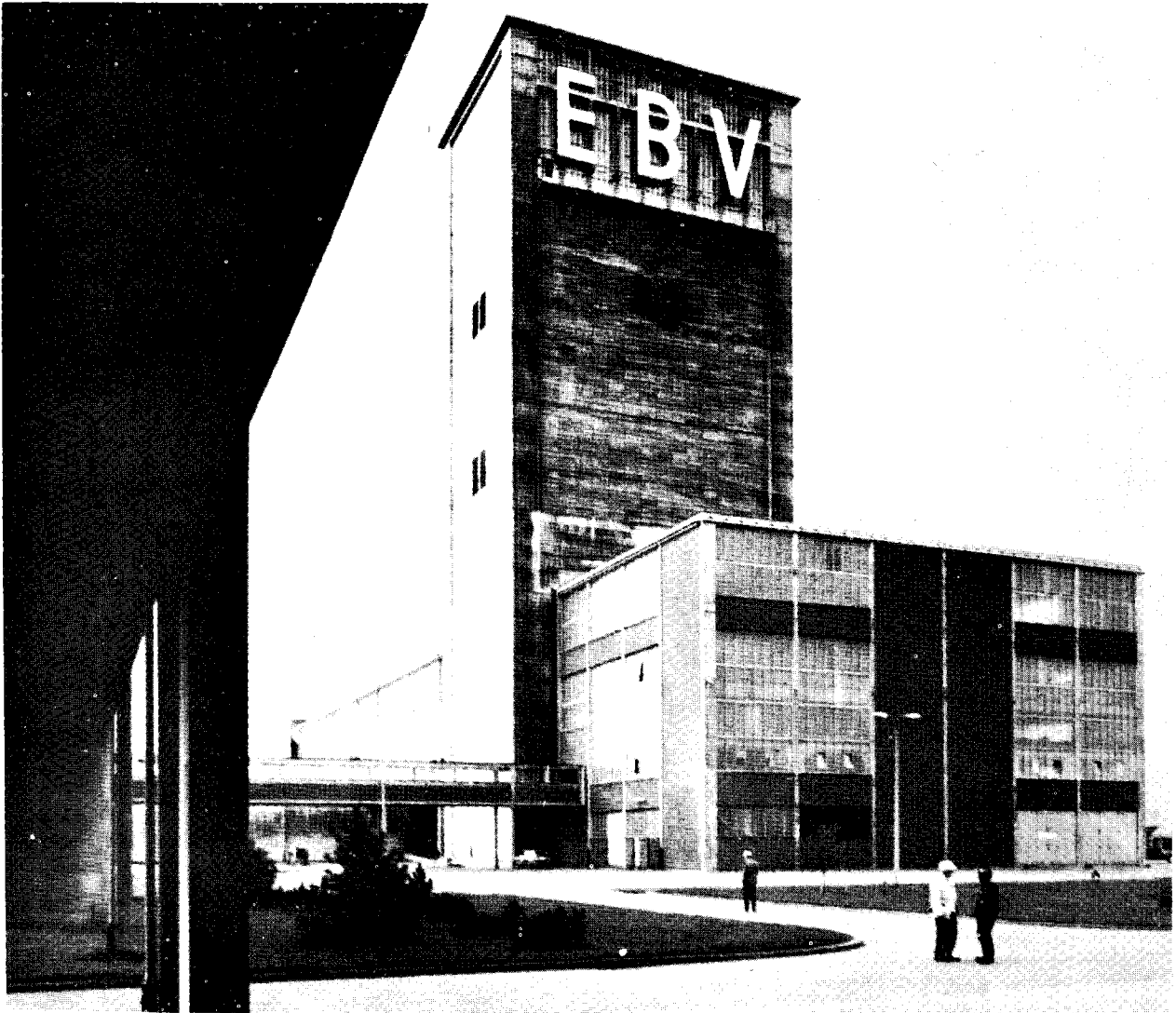
FIGURE 4. - Mine surface structures.
