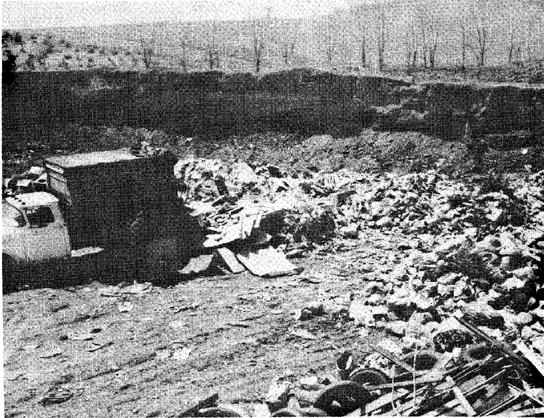
Refuse is discharged from trucks into former strip mine.
