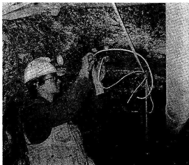
Figure 3.—Geophone installation.
