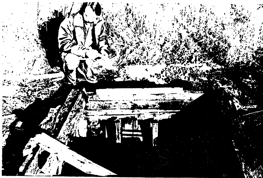
b. Close-up of Warner Mine Air Shaft
