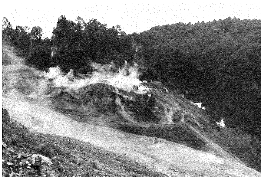
FIGURE 5 - Burning of a Coal Refuse Embankment
