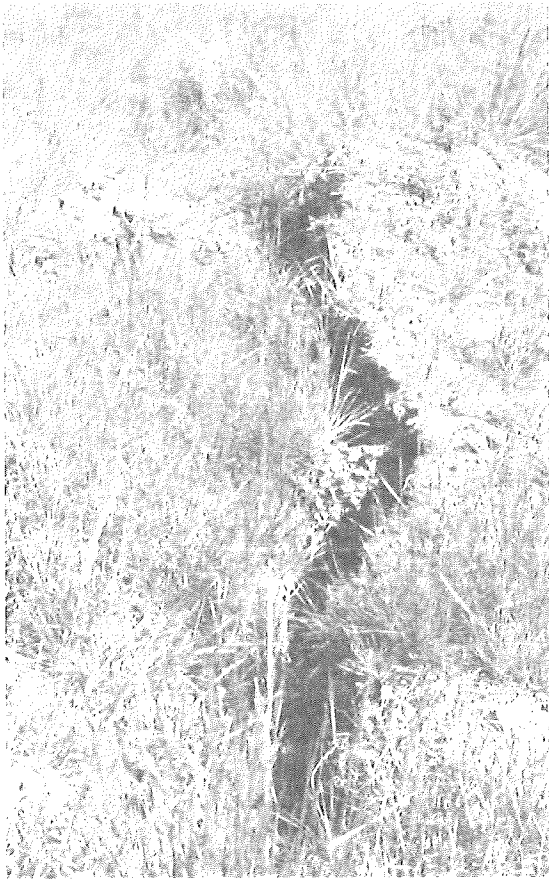
FIGURE 18 - Surface Crack at Roseburg Landslide
