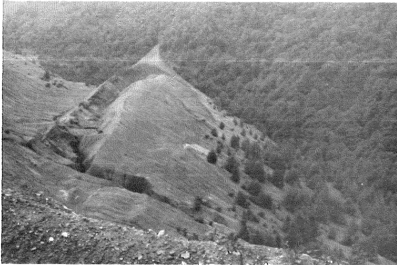
FIGURE 1 - Slope Failure at a Coal Refuse Embankment
