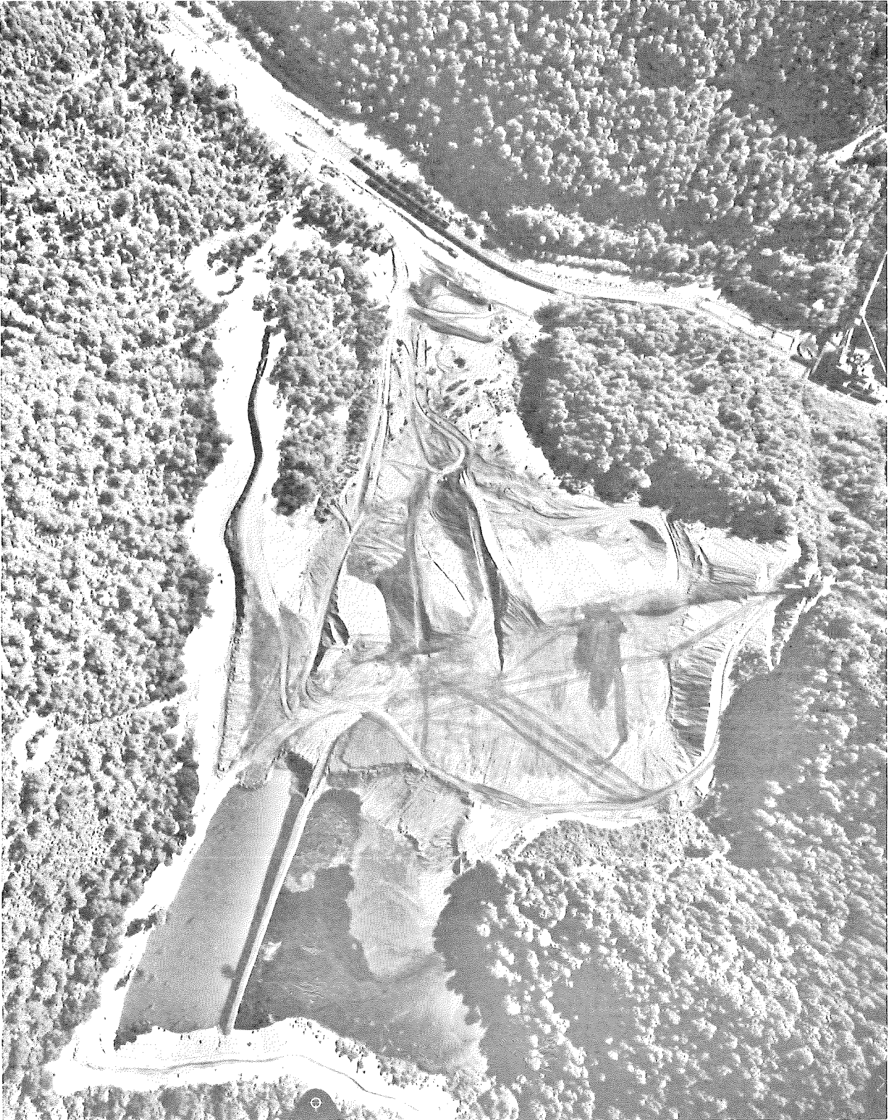
FIGURE 20 - Wharton Refuse Embankment
