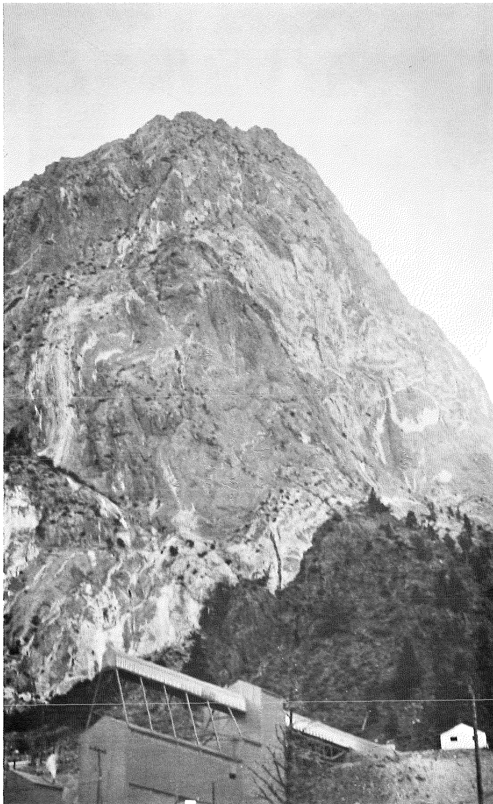
Figure 58 Union Carbide Corporation Pine Creek Mine
