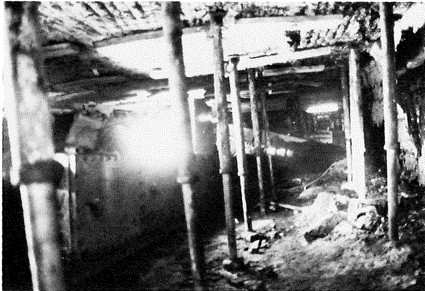
a) HEADGATE AREA
