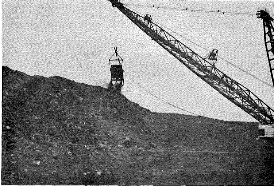
DRAGLINE SPOILING ON THE HIGHWALL
