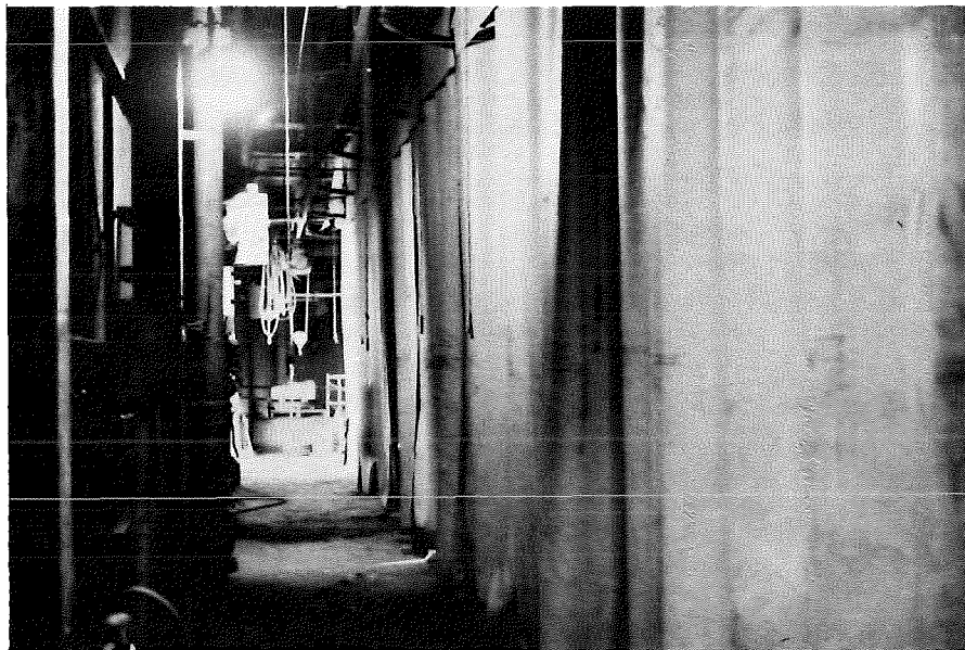
FIG. 74. REINEVELD DRYER AREA AFTER INSTALLATION OF CURTAINS.
