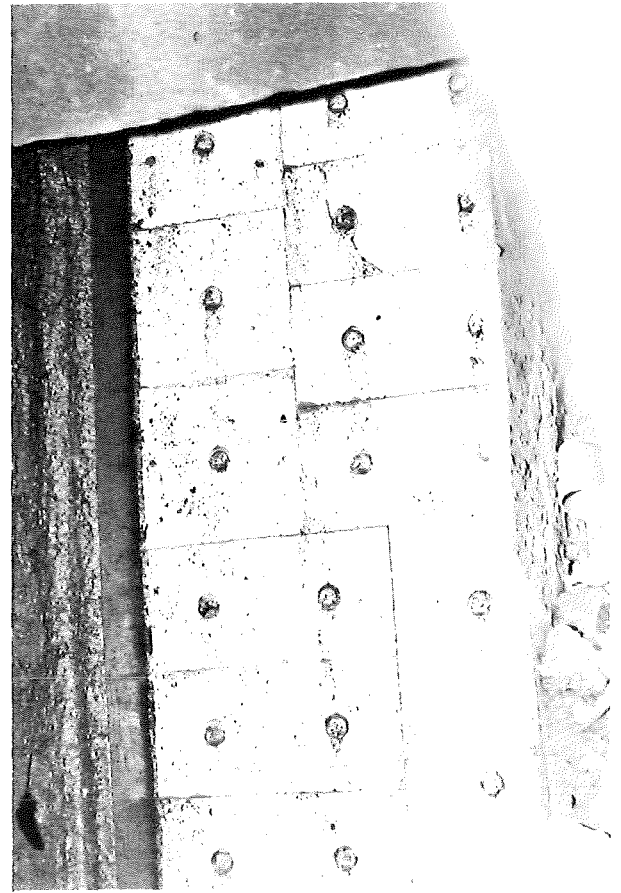
FIG. 46. DURAFLEX CERAMIC TILE INSTALLED IN JIG REFUSE CHUTE.
