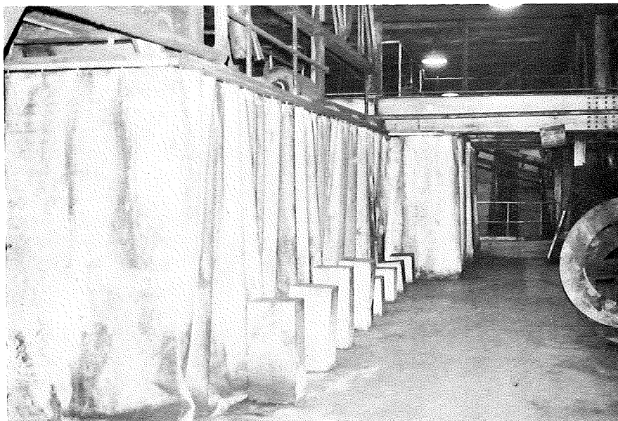
FIG. 61. RIPL-FLO SCREEN FEED CONVEYOR AREA AFTER CURTAIN INSTALLATION.
