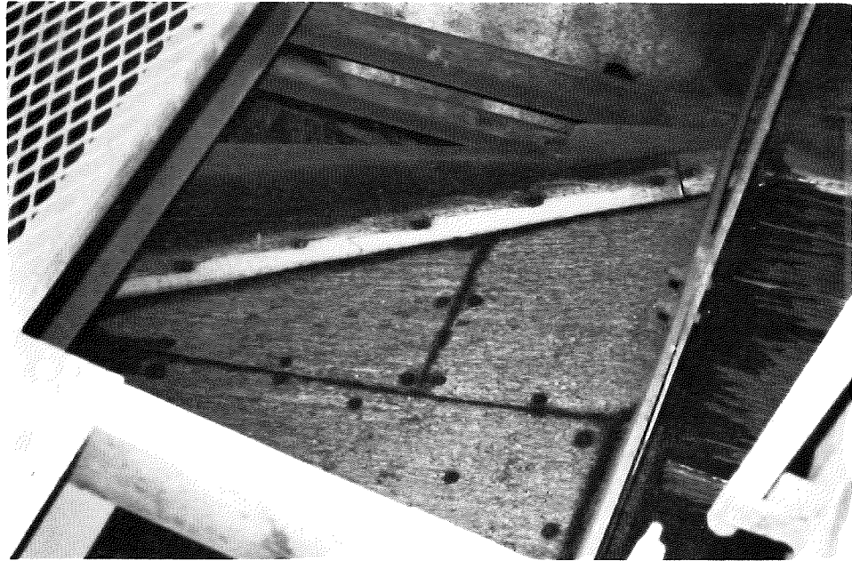
FIG. 38. LINING OF DISCHARGE CHUTES OF SECONDARY SCREEN.
