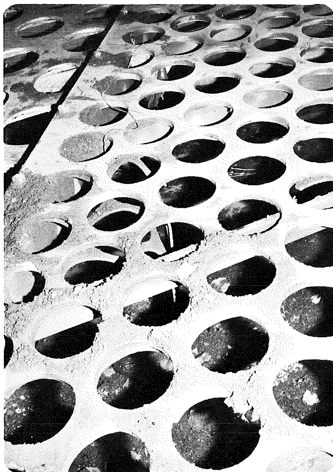
FIG. 22. EAR-DAMPING MATERIAL TORN FROM UNDERSIDE OF STEEL SCREEN (CENTER).
