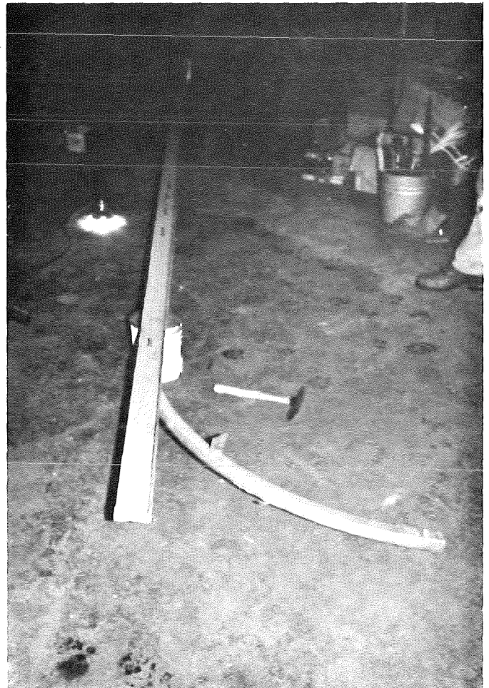
FIG. 42. CURTAIN TRACK BEING BOLTED TO STEEL SUPPORT CHANNEL.
