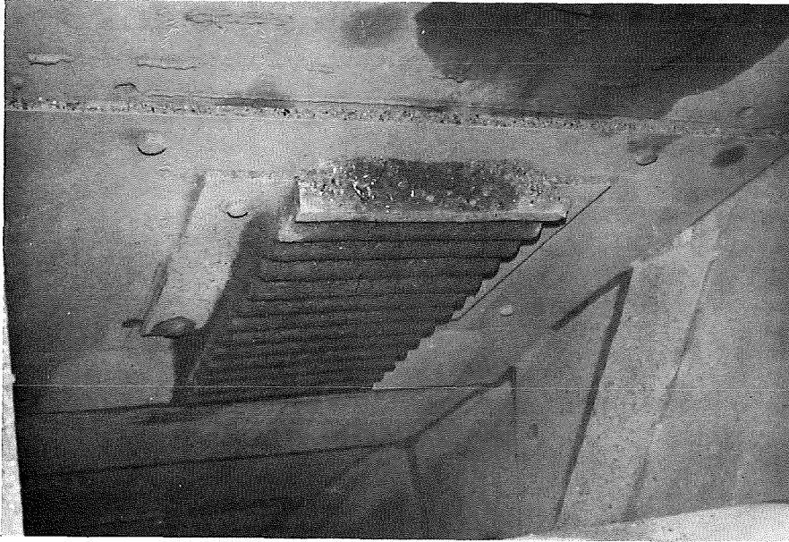
FIG. 77. PROFILED TRELLEBORG INSTALLED AT HEAD END OF CRUSHED COAL BELT (INFEEED TO CLASSIFYING SHAKERS).
