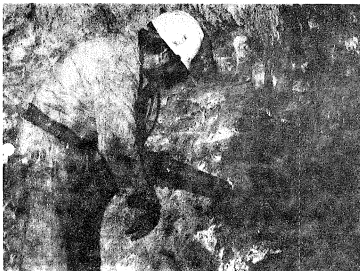
PHOTO OF RIBCLEANSING USING HAND-HELD NOZZLE
