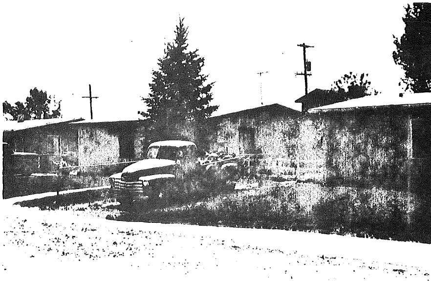
Figure 21. Subsidence over Strathmore mine, South Longmont Street, Yvette. The most recent damage to the street has not yet been repaired. Note unpaved section of street and sagging sidewalk. The coal seam in this area of the Strathmore mine was quite thick, and the probable thickness of coal extracted was 20 to 25 feet. Depth of mining was 100 to 125 feet. Locality 55, subsidence-inventory map.
