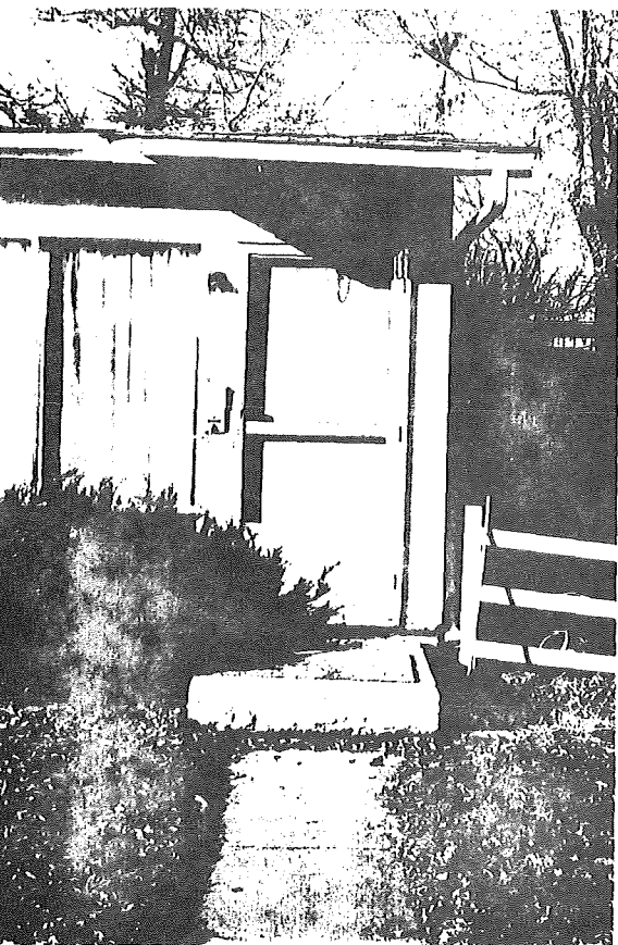
Figure 22. Front stoop of house to the right in Figure 21. This house is immediately south of home shown in Figure 20. The walk has pulled away from the stoop and it in turn has pulled away from the house. Bricks have been jammed beneath the house and beneath the stoop for temporary support. Locality 55, subsidence-inventory map.
