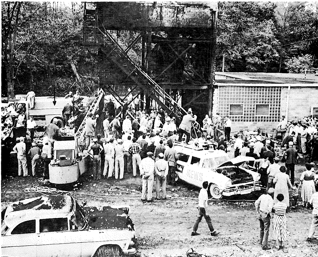
Figure 3. View of Damage to Moore-Shaft Headframe and Truck with Winch and A-Frame After Explosion, Marianna No. 58 Mine, Marianna, Pa., September 23, 1957.
