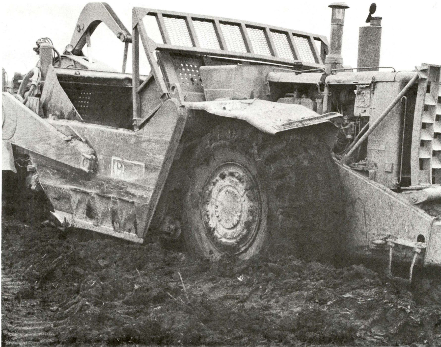
FIGURE 40. PAN SCRAPER LOADING ON MUDDY TERRAIN
