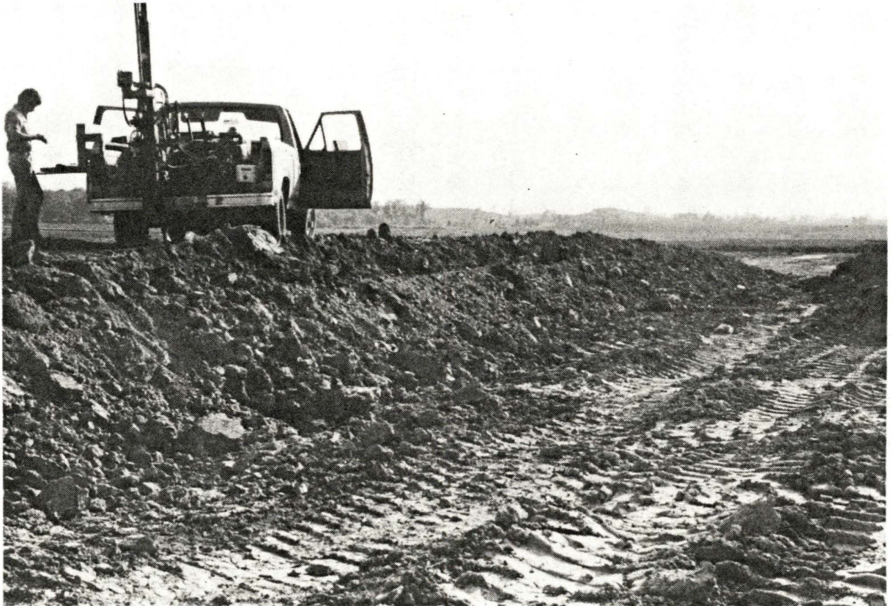
FIGURE 44. Sampling of Fourth Lift of Windrow Test Plot Following Scraper Replacement
