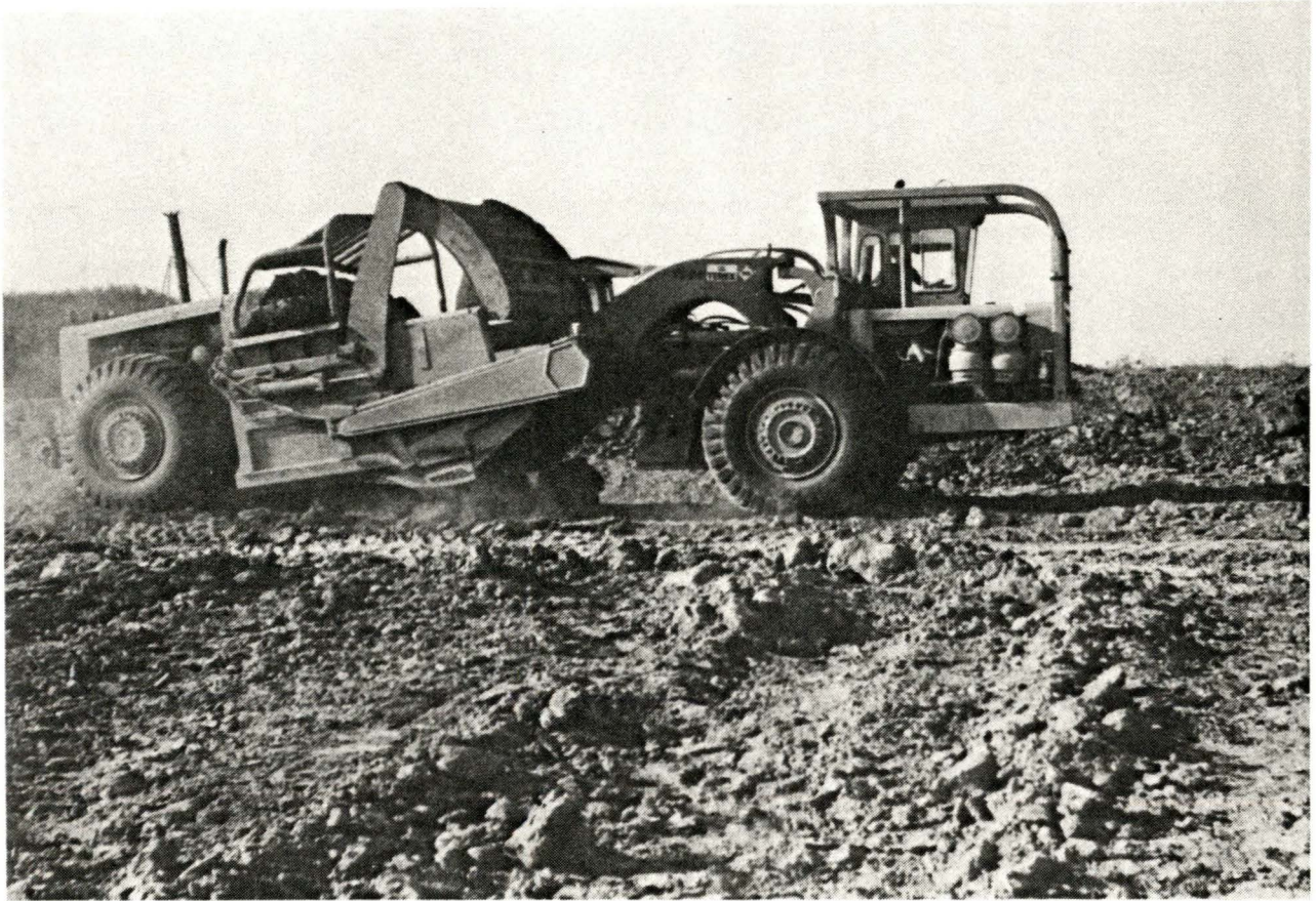
FIGURE 41. Construction of the First Lift of the Scraper Windrow Test Plot with 12 Inches of Subsoil
