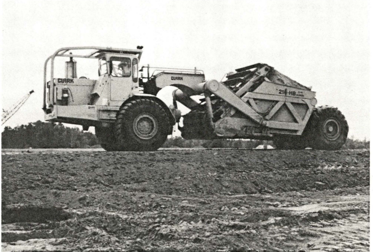
FIGURE 19. Topsoil Windrow Construction on the Brazil Mine
