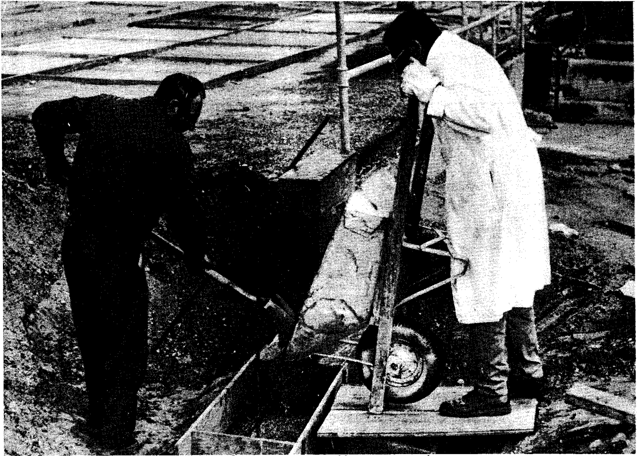
FIGURE 10. - Pouring sulfur concrete footer.
