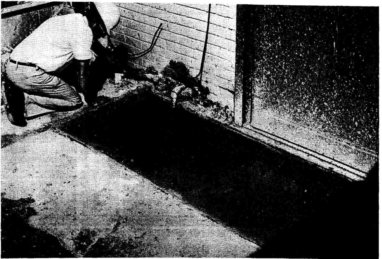
FIGURE 8. - Sulfur concrete paving slab.
