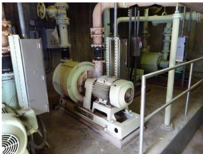
Figure B11. OPS Building 18 basement pumps used for aeration tanks. Photo by NIOSH.
