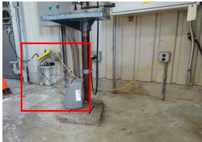
Figure B2. Portable space heater used to keep space warm in Headworks Building 19. Photo by NIOSH.
