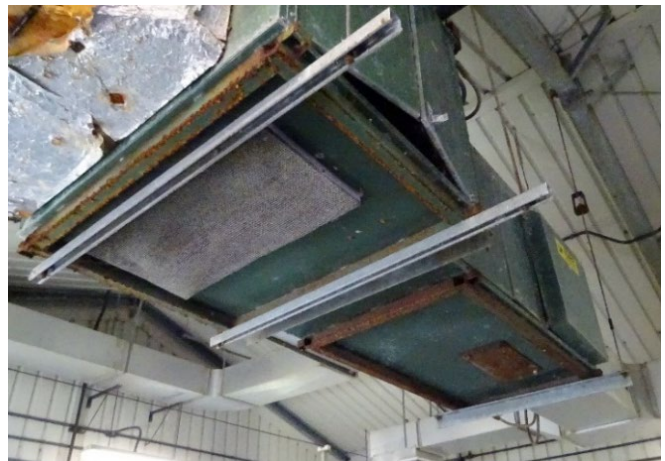
Figure B9. Filter Building 22 ventilation unit over the automated sand filtering banks. Photo by NIOSH.
