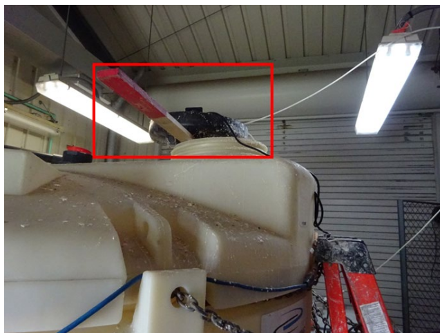
Figure B1. Electric pump for the sludge tank collection. Photo by NIOSH.
