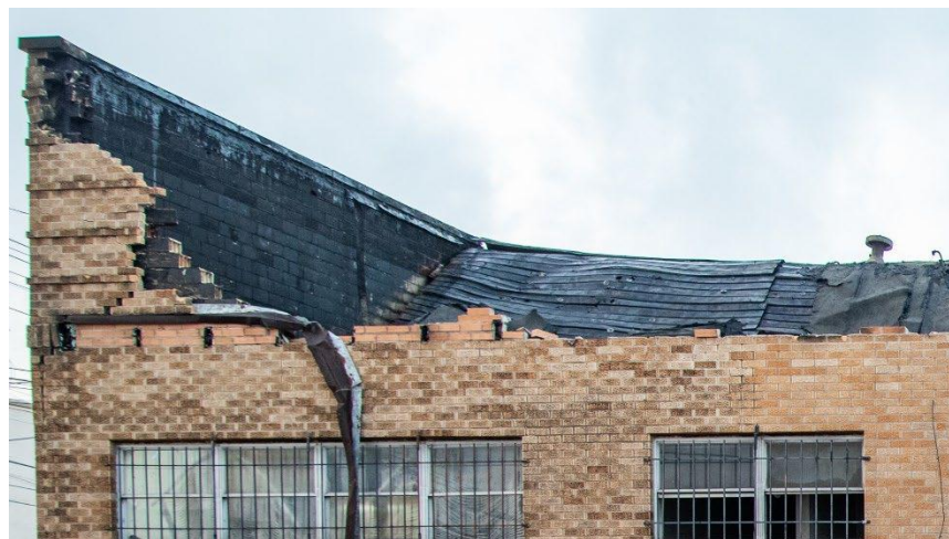
Detail of Delta side wall showing the brick veneer over block wall, slots for previous canopy roof tie ins, roof surface covering. (Courtesy of the fire department)
