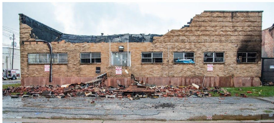
Delta side of structure post-collapse. (Courtesy of the fire department)
