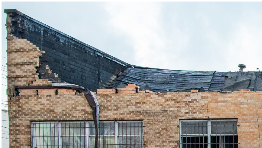
Photo 4: Detail of Delta side wall showing the brick veneer over block wall, slots for previous canopy roof tie ins, roof surface covering. (Courtesy of the fire department)
