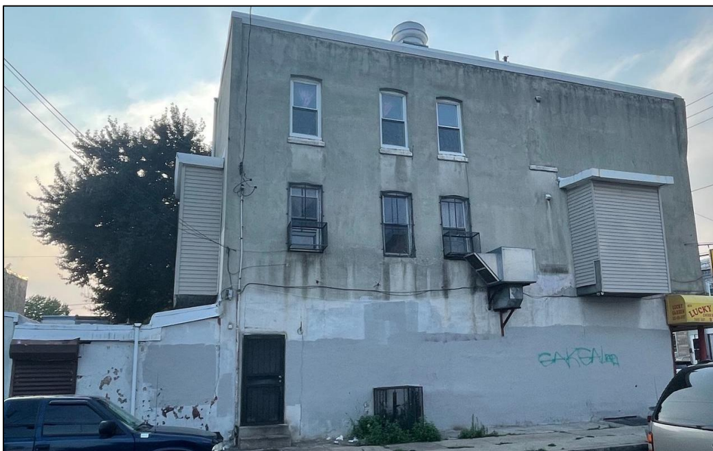
Photo 3: Bravo side of the structure. Note the bump out over the sidewalk and exposed windowsills where windows were covered over. (Courtesy of fire department)
