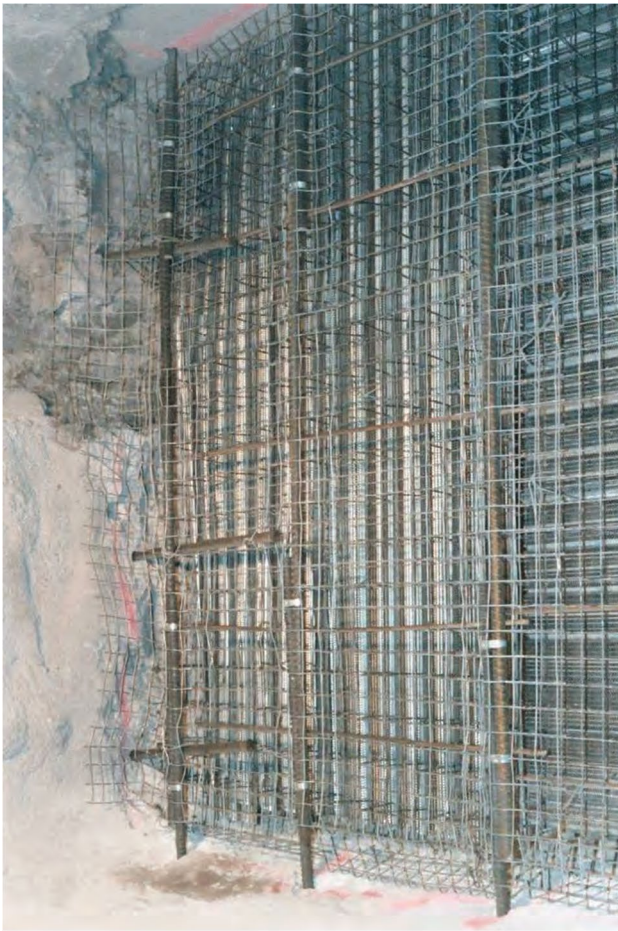
Fig. 6 The rear Insteel panel with Stayform backing, one plane of vertical #8 steel reinforcement bars and anchors, the horizontal #8 steel reinforcement bar anchors, and the horizontal #3 steel reinforcement bars are seen in this Insteel 3D seal under construction [4]
