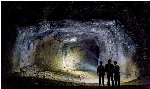
Fig. 3 Excessive spillage of clayey material and water from an open karst void [5]
