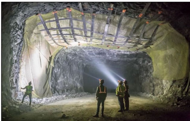
Fig. 4 Ground support measures taken around Pillar-X [4]
