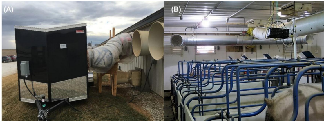
Figure 2. Ductwork installed in the treatment room: (A) outside attached to air handling unit and (B) inside the treatment room.
