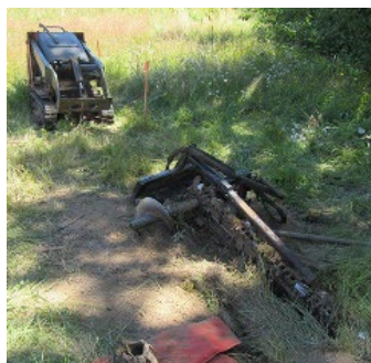
Mini skid steer with trencher attachment.
