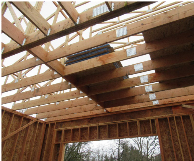
View through the unfinished floor of the room above the garage. The leading edge of the floor is on the right and the OSB sheathing is stacked on floor joists.
