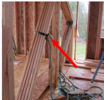
Example of how crew tied-off lifeline ropes to roof trusses.
