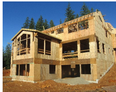
House where framer fell 25 feet from the lower back sheathed roof. He was not using fall protection.
