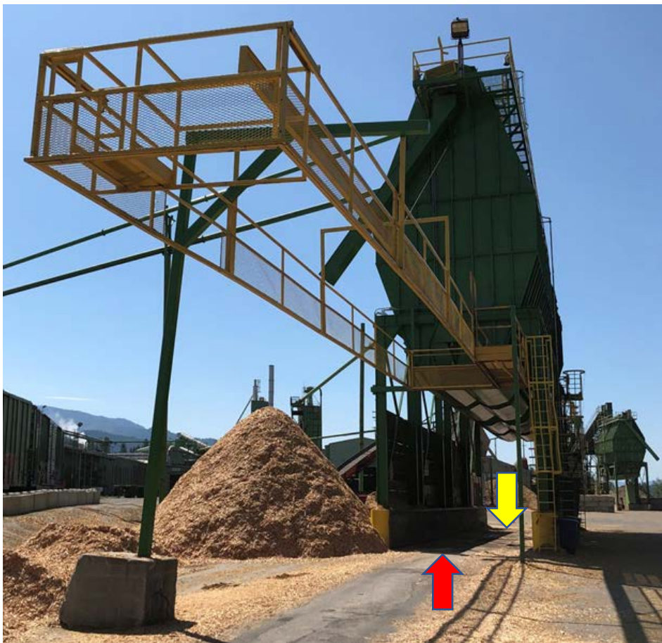
Photo 10: Red arrow shows where the back of the fatally injured driver's trailer was located under the tarping station. Yellow arrow shows where the front of the second truck's tractor was located under the bins when the incident occurred. Approximately 30 feet of space separated the trucks. The road under the tarping station had a 2% downward grade toward the exit.
