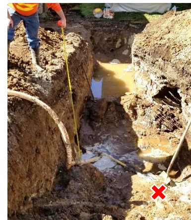
Unprotected trench after its sidewall collapsed. The "x" indicates the laborer's location.
