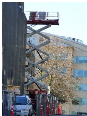
Incident scene showing the scissor lift from which the laborer fell 60 feet.
