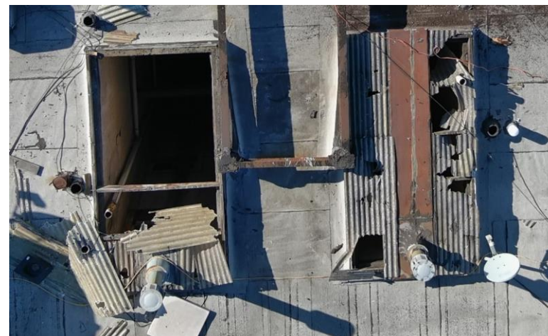
View of the two light/air shafts with removal of panel (south shaft) and ventilation holes (north shaft). (Photo courtesy of Fire Marshal's Office)
