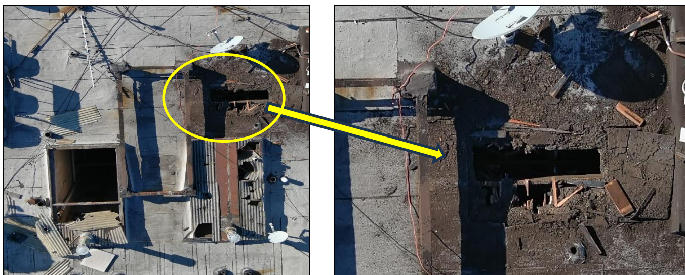
Photo 8 and Photo 9. View of ventilation hole (Photo courtesy of Fire Marshal's Office)
