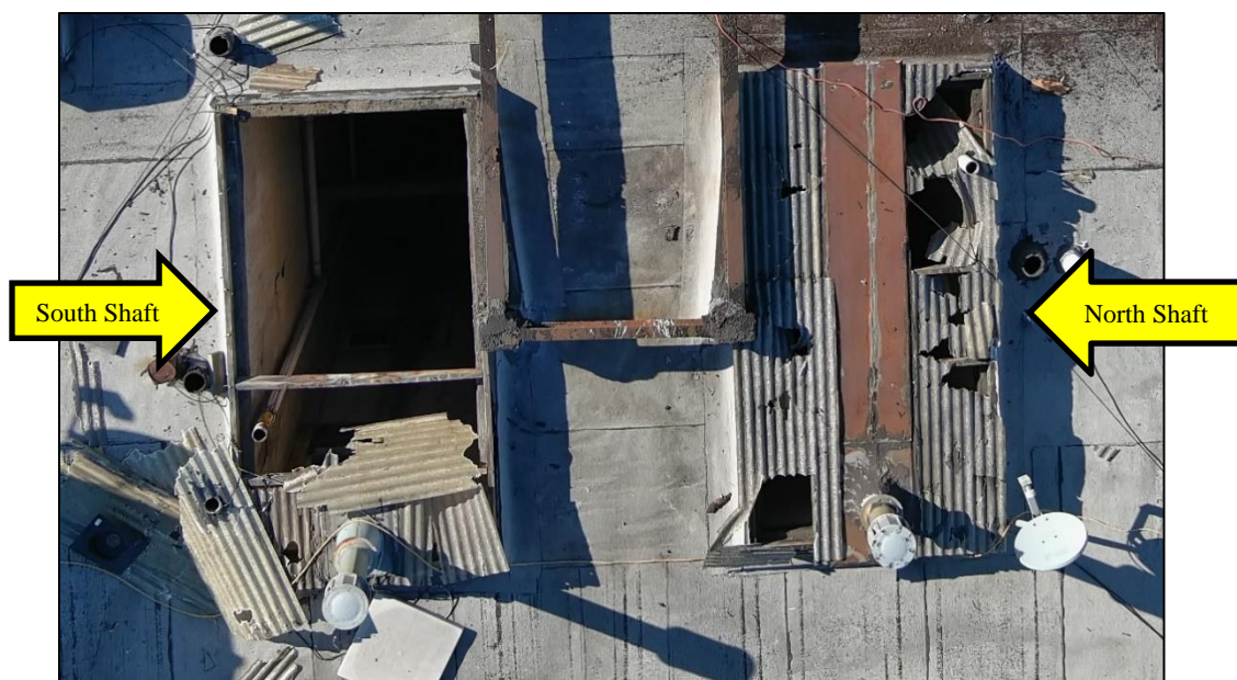
Photo 7. View of the two light/air shafts with removal of panel (south shaft) and ventilation holes (north shaft).
